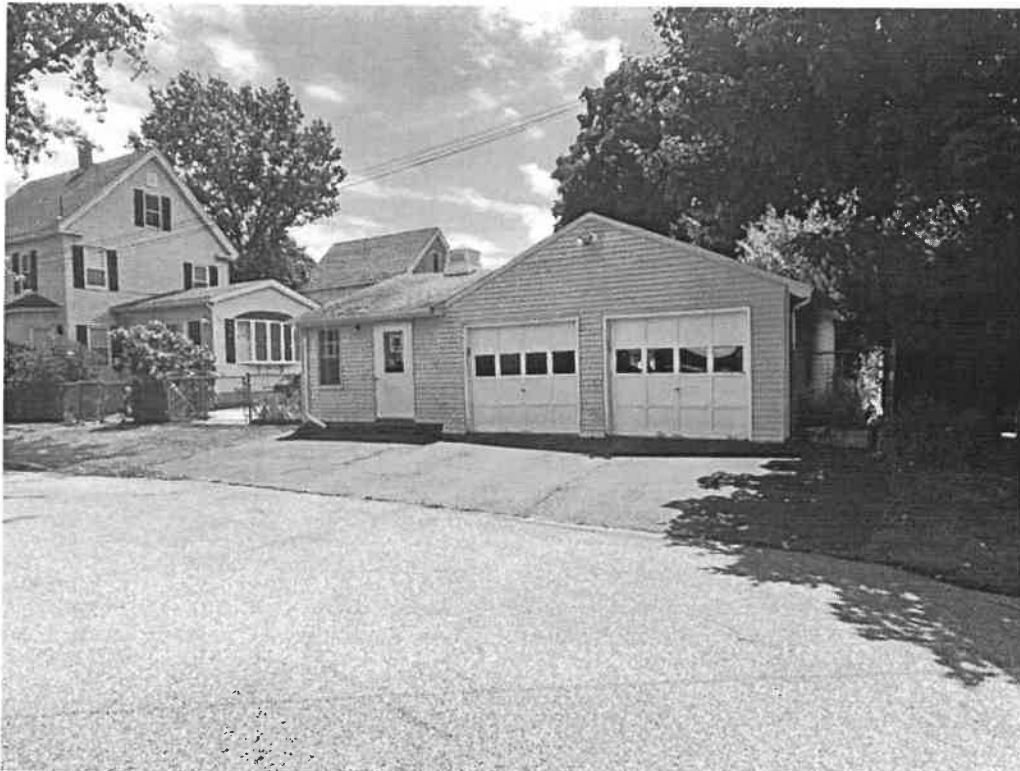
3. 294 Thornton St. (across-Whipple neighbor without req'd side nor front setback)
