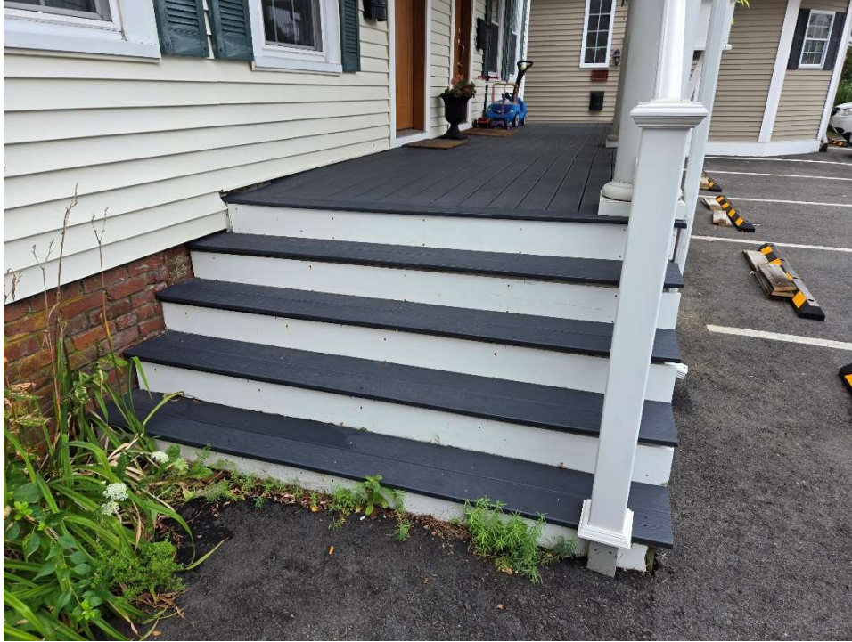
Existing stairs, left side, 962 Islington
