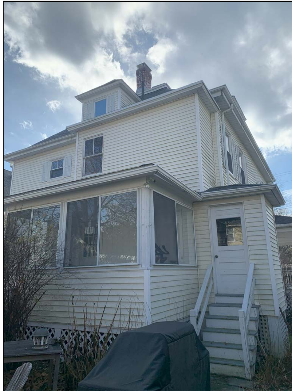
VIEW FROM REAR OF DRIVWAY LOOKING SOUTH
