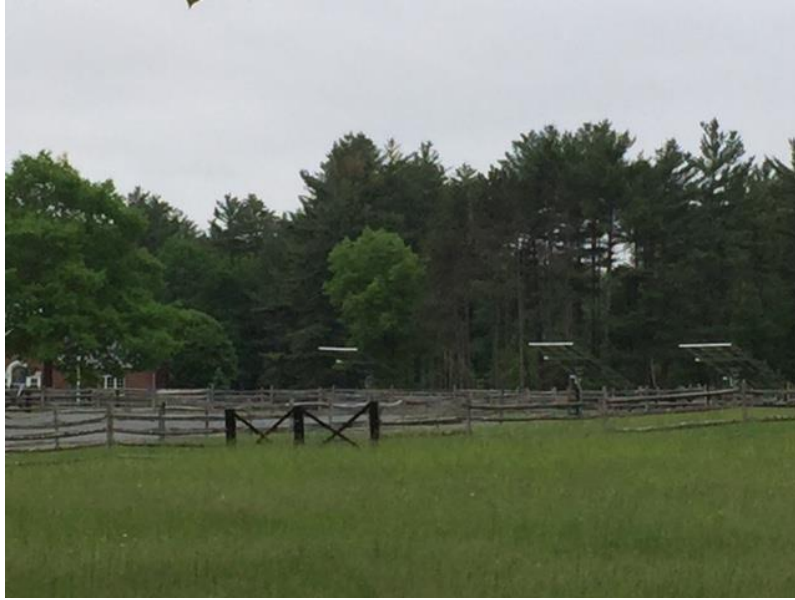
Pole mounted system – agricultural site.
