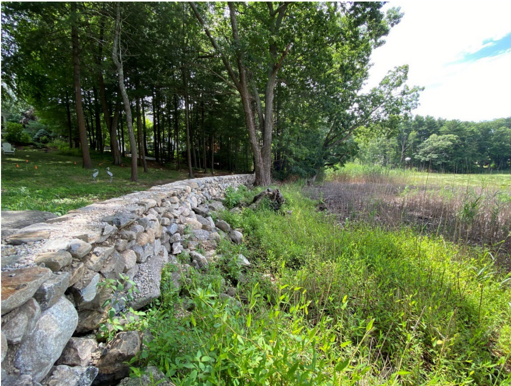
Photo 8. Overview of the downslope side of the stone wall, viewing south from the northern end of the stone wall. Wetland POGW1 occurs in the right side of the photo. (08-11-22)
