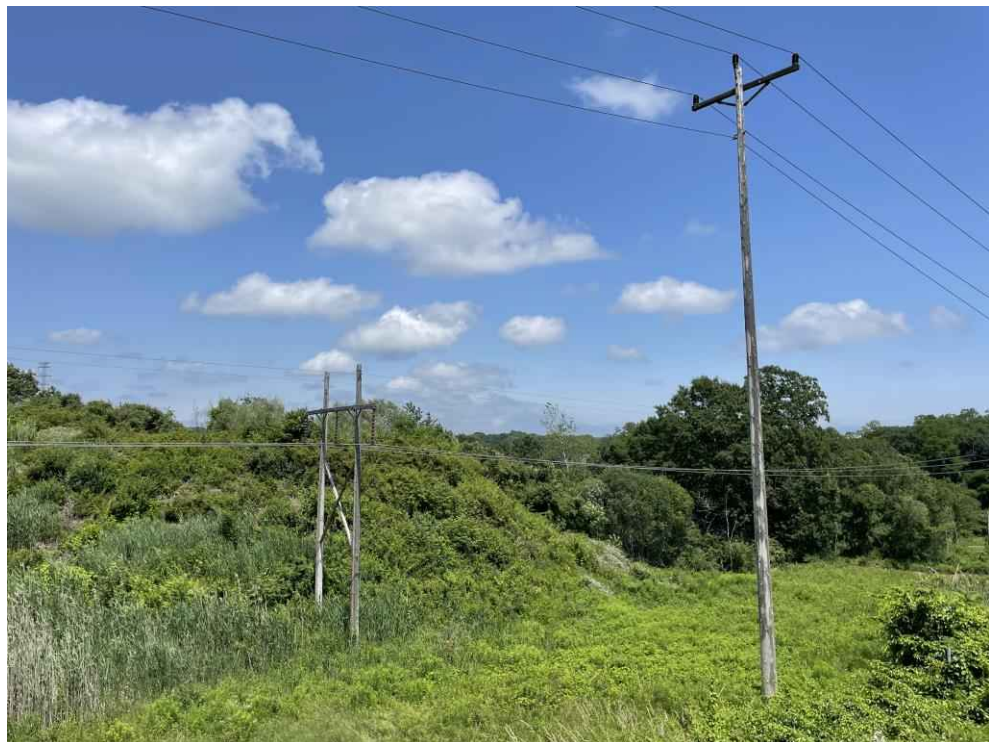
Photograph No. 34: Looking northeast at Structure 9 and Wetland PW-12 (PEM1/PSS1E) on the T13 Line ROW off Gosling Road, Portsmouth, NH.
