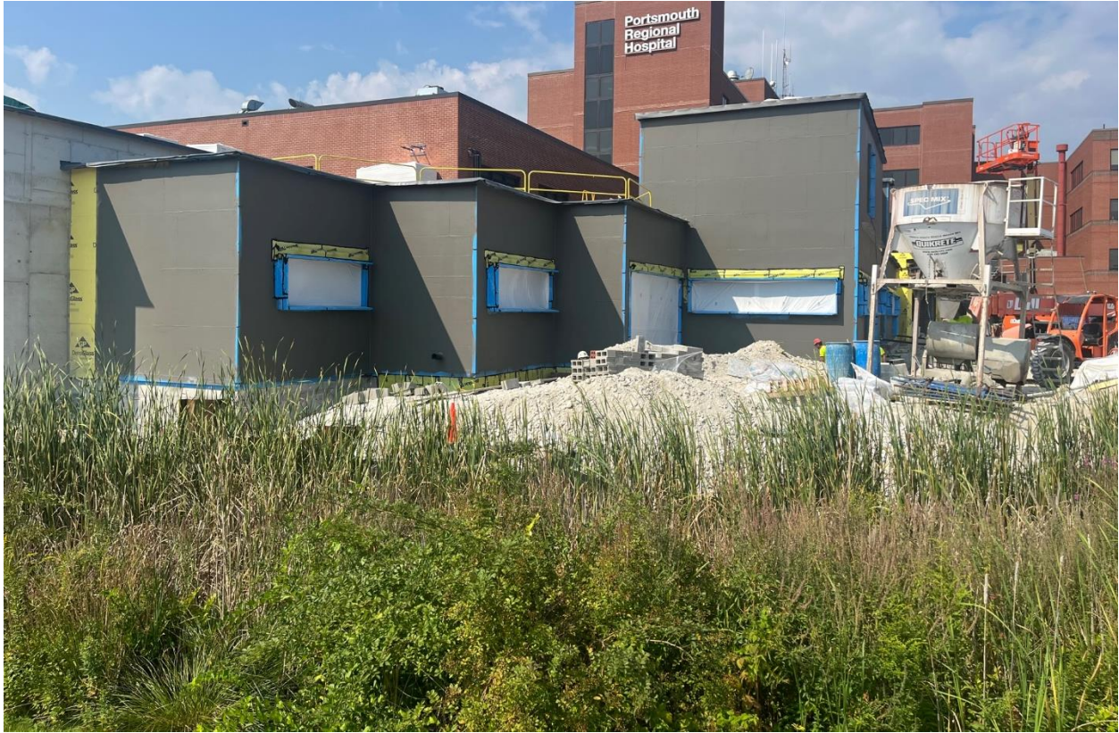
Photo #5: Looking at the almost finished exterior of the ongoing construction.
