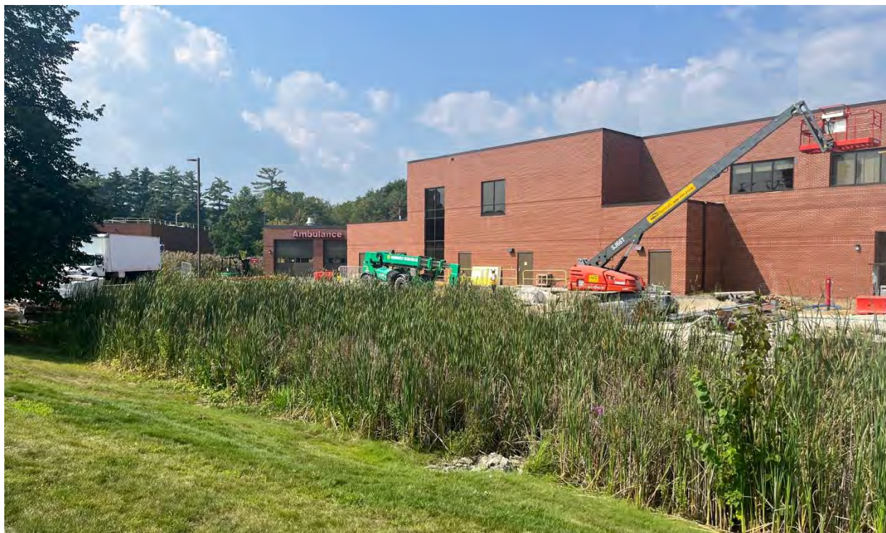
Photo #3: Looking at the construction activities from Borthwick Ave.
