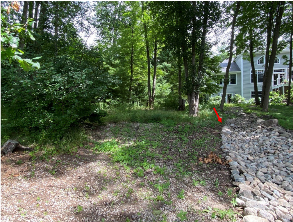
Photo 30. Lower portion of wetland POGW2, viewing east upslope from near the bottom of the stone swale. Top of the stone swale extension is indicated by the red arrow (08-11-22)
