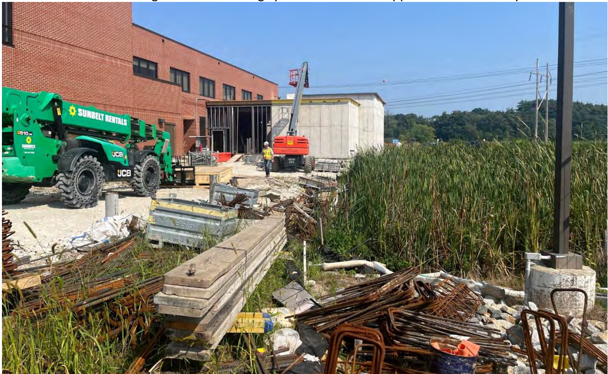
Photo #2: Looking at the continued construction at the location of the mobile unit.
