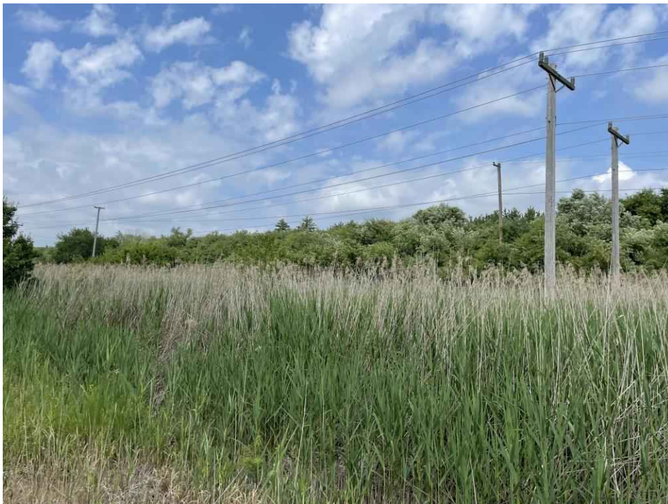
Photograph No. 14: Looking west at Wetland PW-1 (PEM1/PSS1E.Fg) near Structure 81 on the 3171 Line ROW off NH33, Portsmouth, NH
