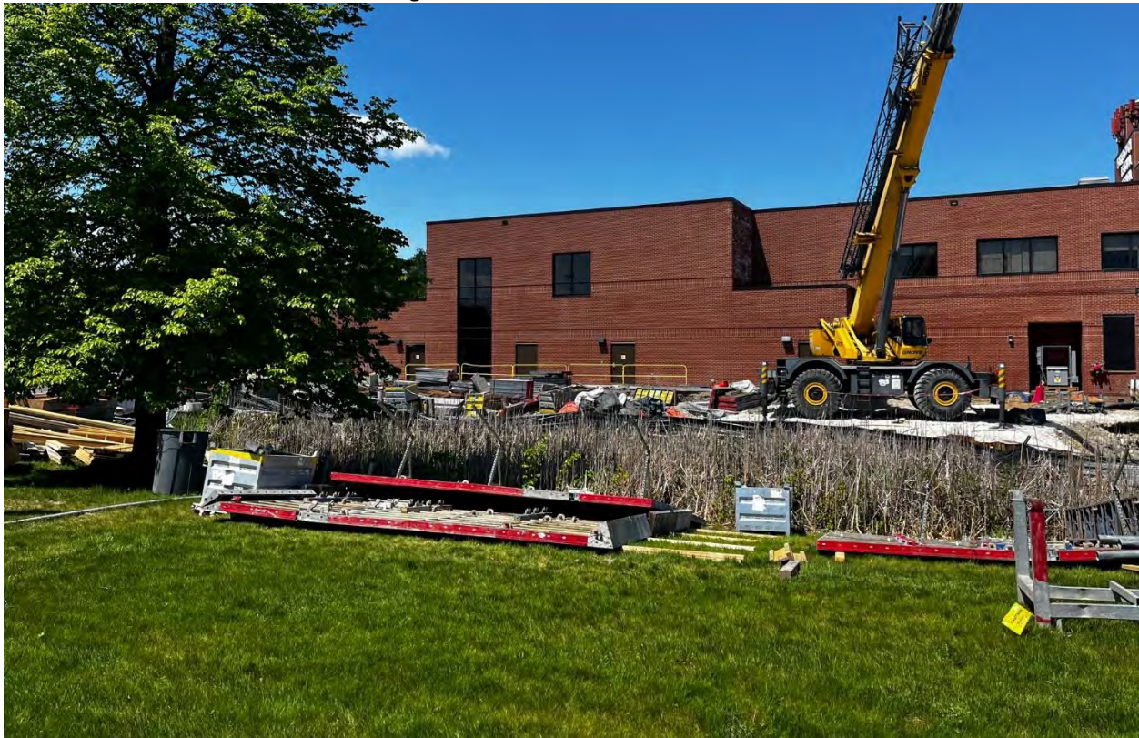
Photo #4: Looking at the active construction area.
