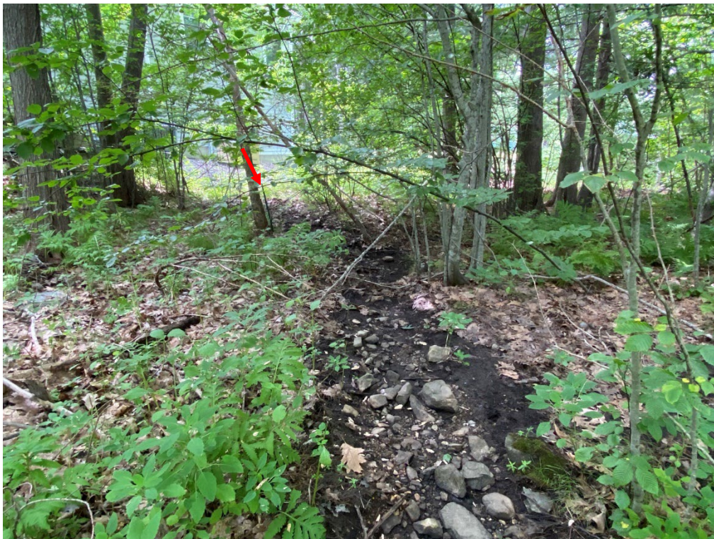
Photo 20. POGS1 leading onto the Gardner property from the culverts located at the northeastern end of POGW2, viewing south, downstream. Property boundary is indicated by the green rod indicated by the red arrow. (08-11-22)
