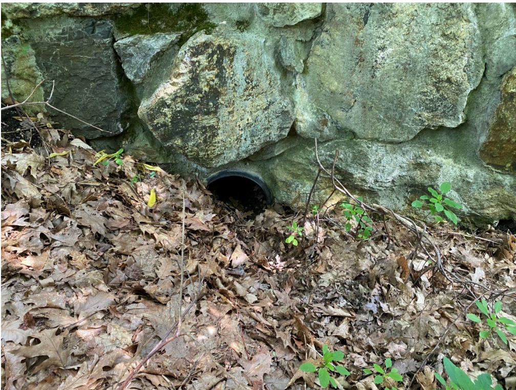
Photo 16. Northern culvert outflow (source of delineated POGS2) into POGW2, viewing west. (08-11-22)
