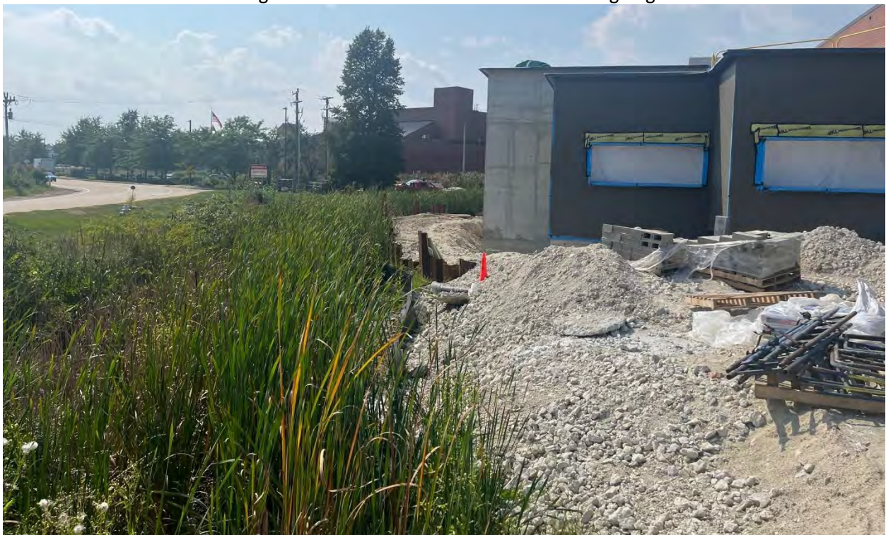
Photo #6: Looking at the ongoing construction and stable erosion control methods.
