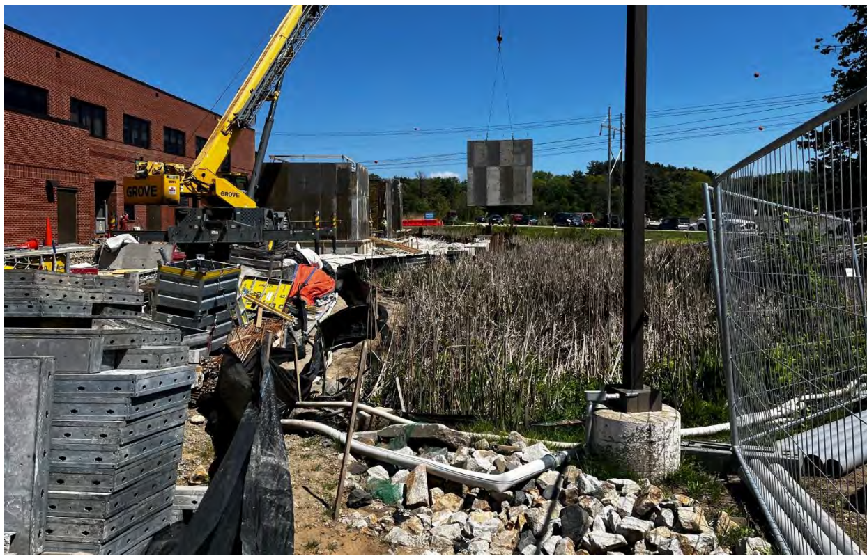
Photo #9: Looking at the ongoing construction and erosion controls.
