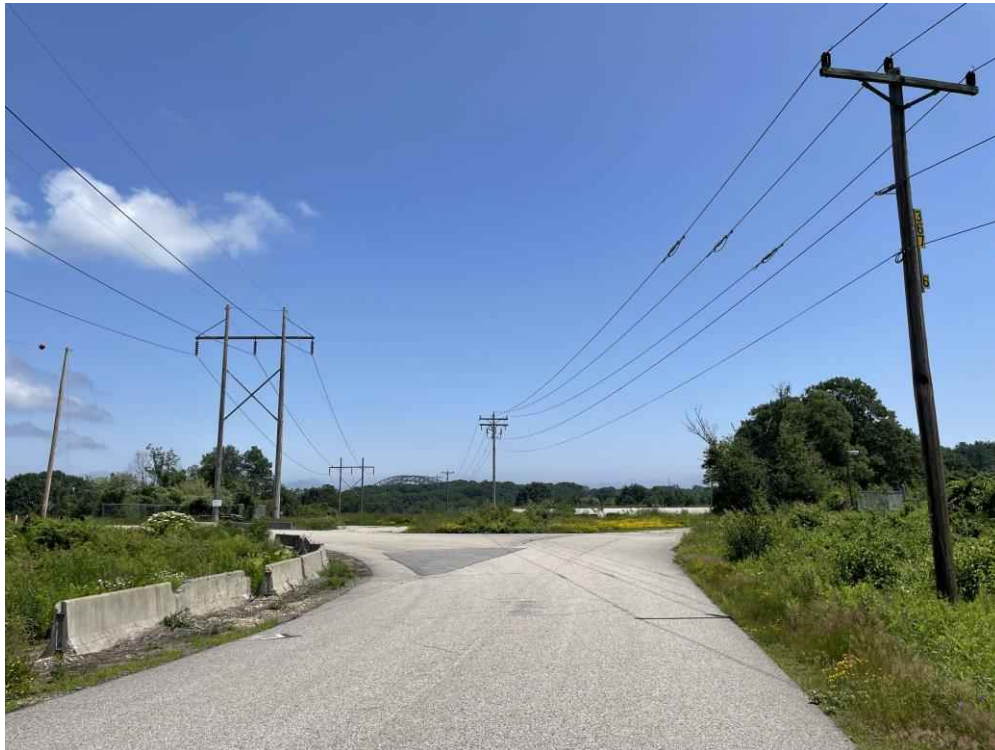
Photograph No. 32: Looking east at Structure 7 and Wetlands PW-10 (PSS1Ex) and PW-11 (PSS1/PEM1Ex) on the T13 Line ROW off Gosling Road, Portsmouth, NH.
