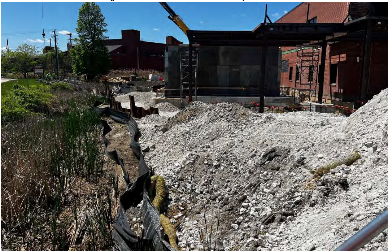
Photo #8: Another view of the erosion control measures.
