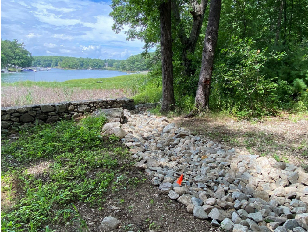
Photo 31. Bottom of the new portion of the stone swale, viewing west. (08-11-22)
