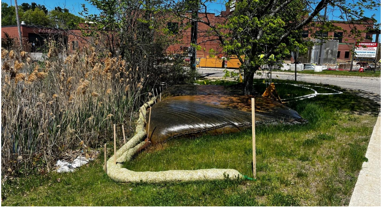
Photo #1: Looking at the dewatering area for the project.
