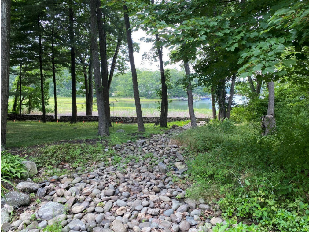
Photo 27. Overview of the older portion of the stone swale, viewing west from the near the top of the swale. (08-11-22)
