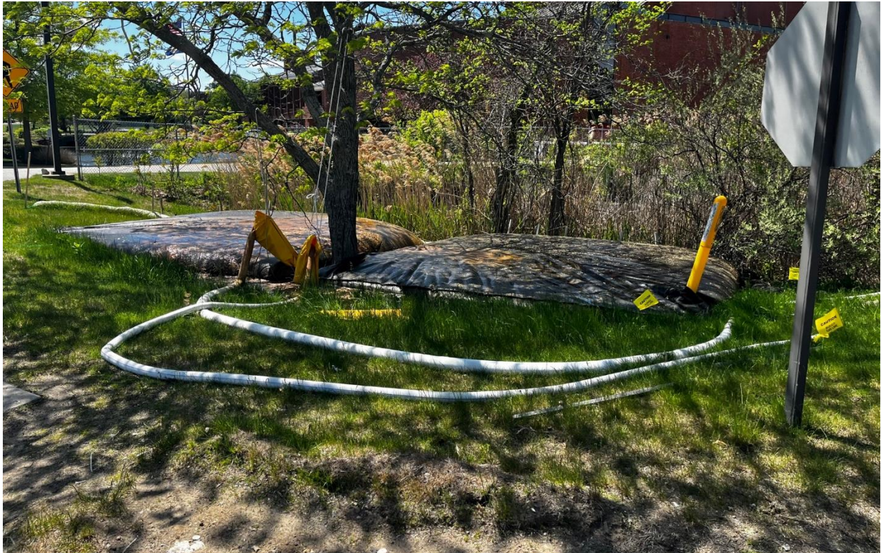
Photo #2: Another view of the dewatering system.
