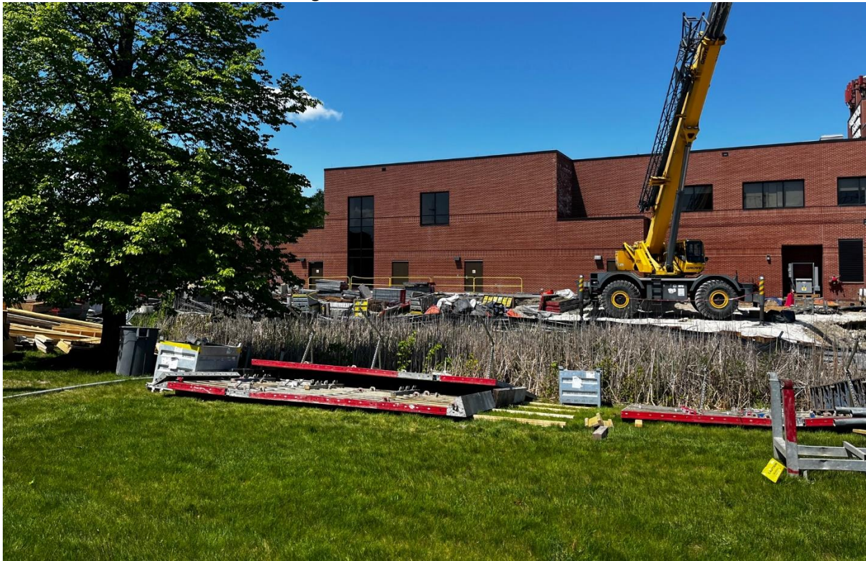
Photo #4: Looking at the active construction area.
