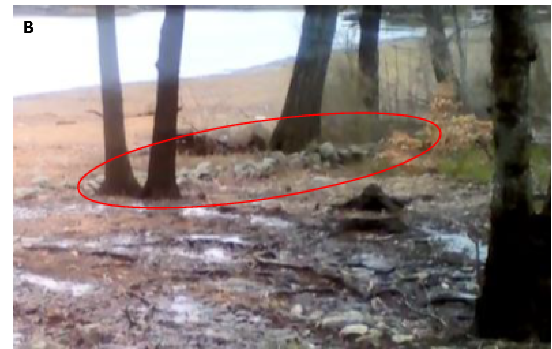
FIGURE 2. A) SCREEN CAPTURE FROM VIDEO SHOWING CONDITIONS ON IN VICINITY OF THE CURRENT LOWER HALF OF THE SWALE. VIDEO DATES TO PRIOR TO THE STONE WALL REBUILD IN 2022 BUT AFTER THE COMPLETION OF THE UPPER STONE SWALE INSTALLTION IN 2017. AREA CIRCLED IN RED REPRESENTS THE SECTION OF UNDISTURBED STONE WALL TO SERVE AS THE TEMPLATE FOR THE STONE WALL RESTORATION BASED ON DISCUSSIONS WITH THE CITY AND NHDES. B) ZOOMED IN VIEW OF THE TEMPLATE SECTION OF STONE WALL
