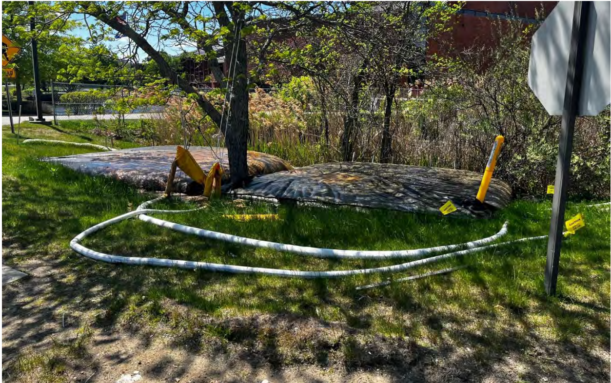
Photo #2: Another view of the dewatering system.
