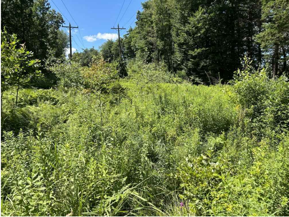
Photograph No. 11: Looking east at Structures 85 and 84 on the 3171 Line ROW off NH33, Portsmouth, NH
