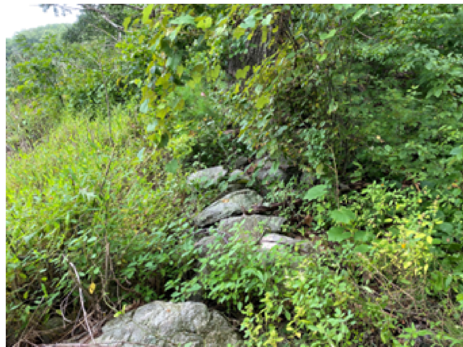
FIGURE 1. UNDISTURBED PORTION OF STONE WALL AT NORTHERN END OF PROPERTY. CORRESPONDS WITH THE SECTION OF STONE WALL CIRCLED IN RED IN FIGURE 2. (8/26/23)
