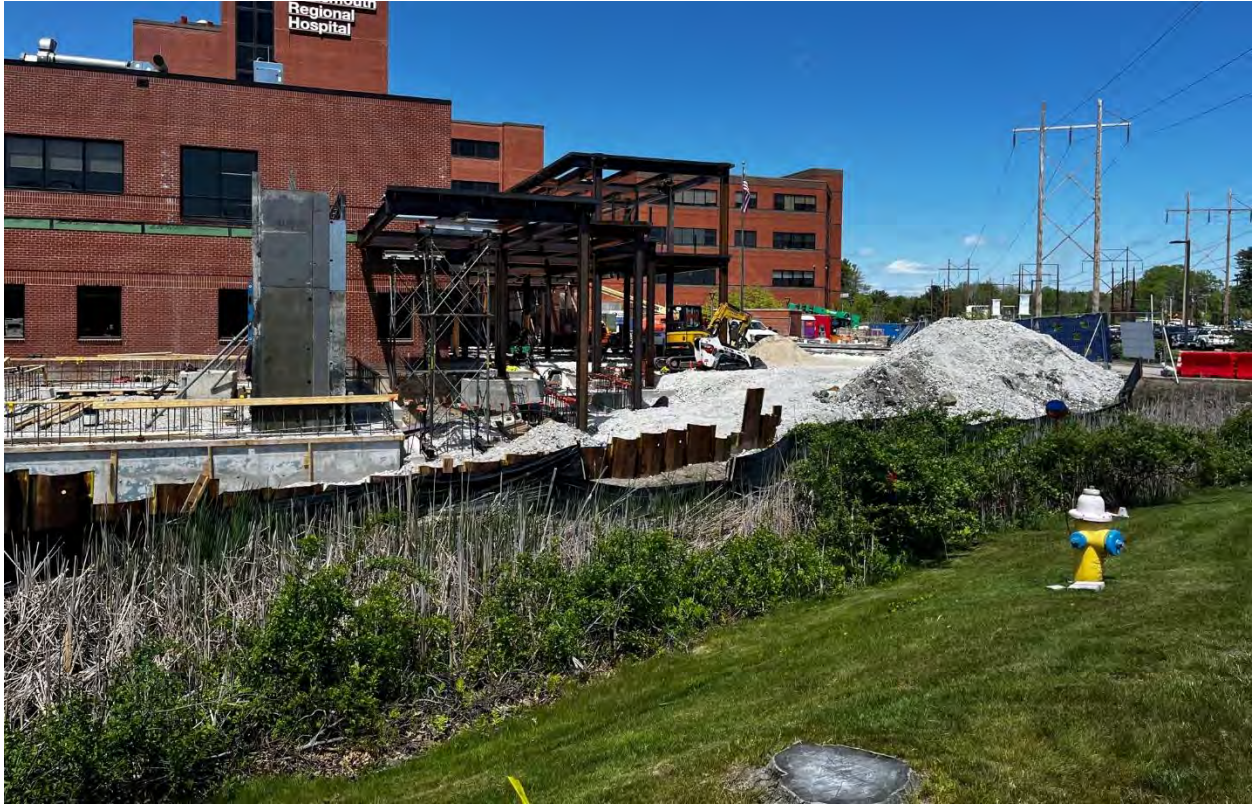
Photo #5: Looking at the ongoing construction and erosion control.
