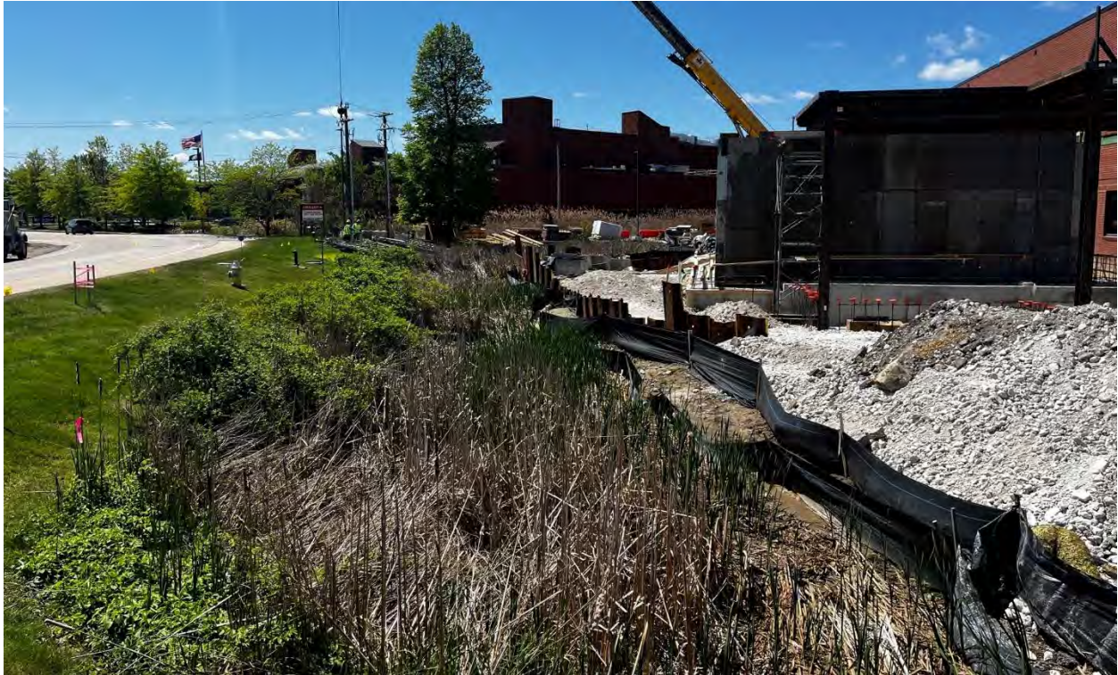
Photo #7: Looking at the erosion control methods adjacent to the construction.
