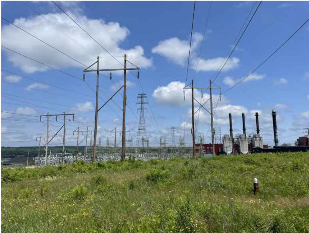
Photograph No. 19: Looking northeast at Structure 1 on the T13 Line ROW off Gosling Road, Portsmouth, NH.
