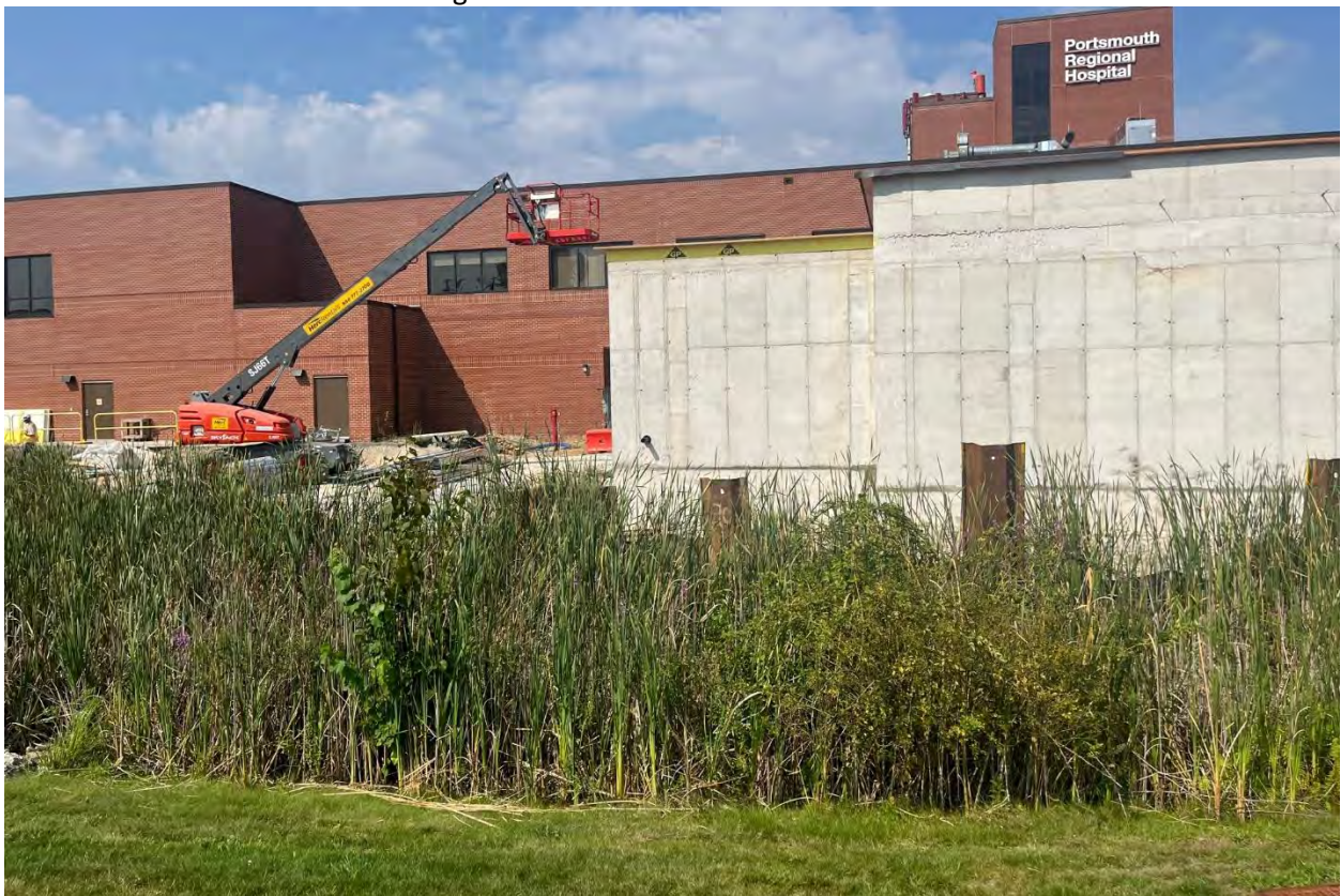
Photo #4: Looking at the almost complete exterior structure.
