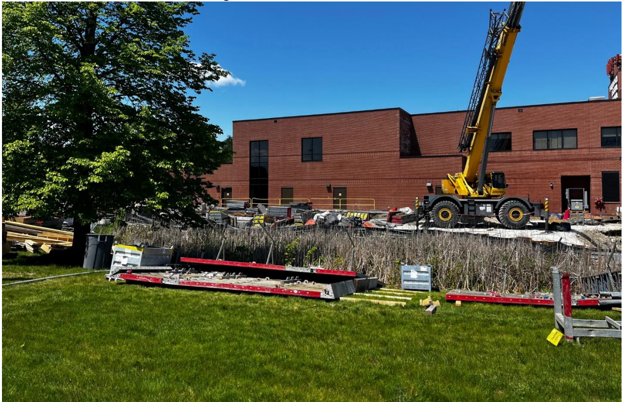
Photo #4: Looking at the active construction area.
