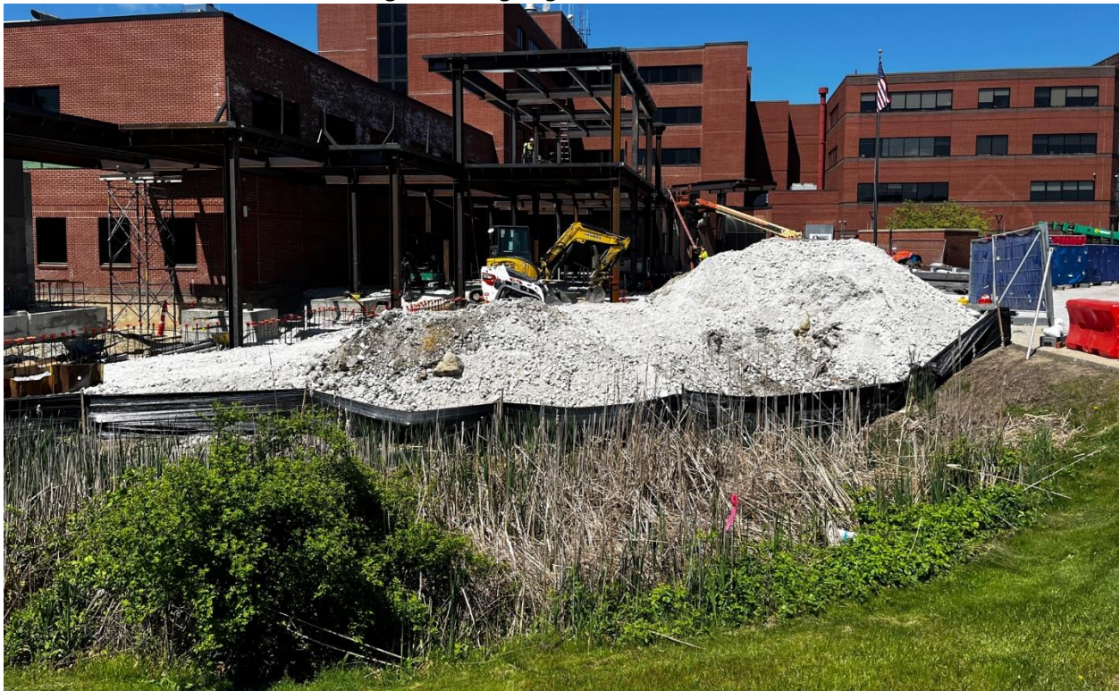
Photo #6: Looking at the ongoing construction and erosion controls.
