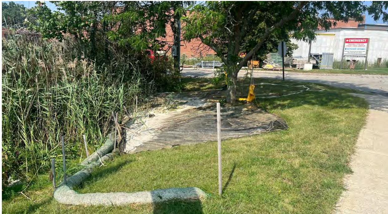
Photo #1: Looking at the dewatering system that doesn't appear to be in use anymore.
