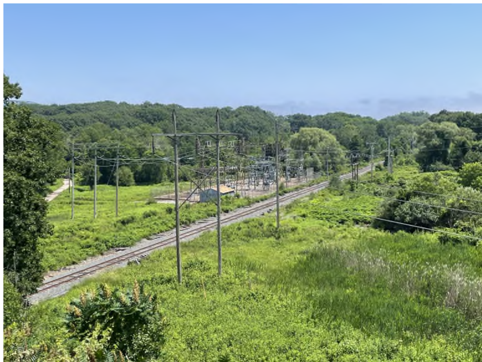
Photograph No. 34: Looking southeast at Wetlands PW-13 (PEM1/PSS1E), PW-14 (PSS1/PEM1E), and PW-15 (PEM1E), and at Structures 10 and 11 on the T13 Line ROW off Gosling Road, Portsmouth, NH.
