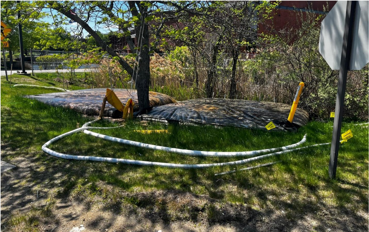
Photo #2: Another view of the dewatering system.
