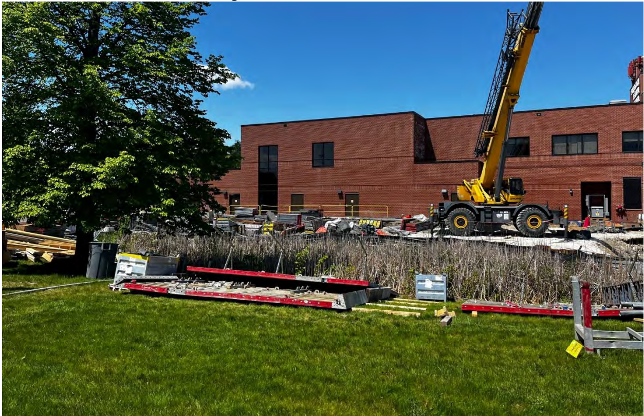
Photo #4: Looking at the active construction area.
