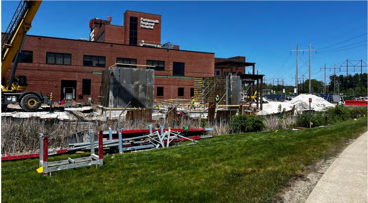
Photo #3: Looking at the construction area from Borthwick Ave.
