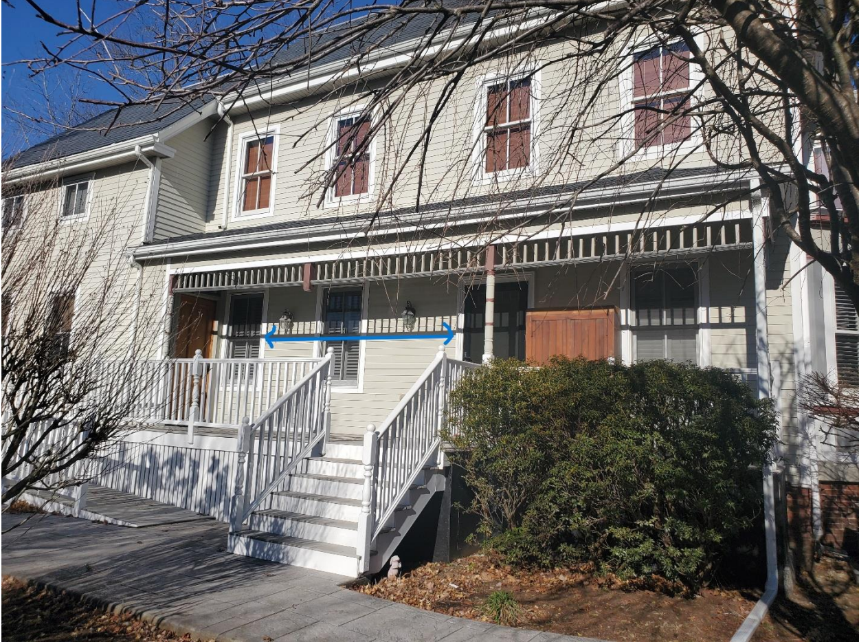
Side of condo. Door and window to be switched.
