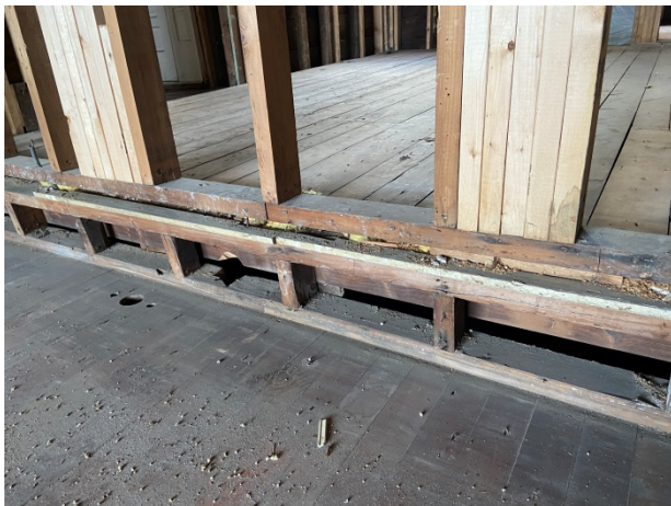
25-Post bearing on short studwall
