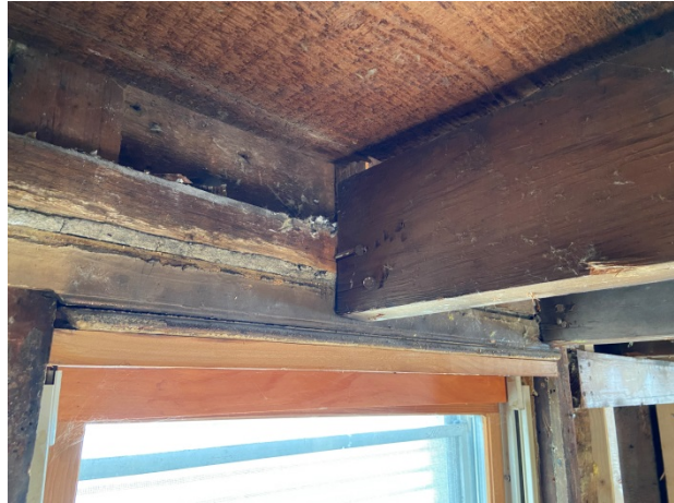
28-Joist connection to wall framing
