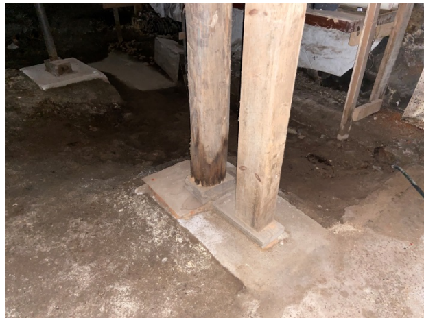
14-Detail of typical wood post bearing
