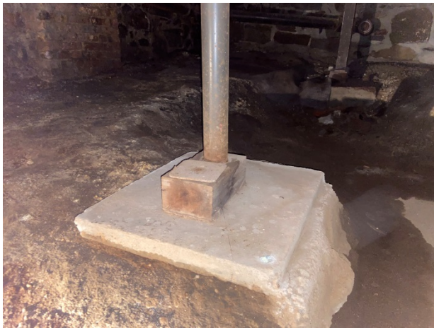
13-Detail of screw jack bearing on wood
