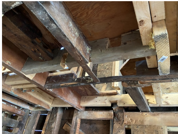
20-Front bay second floor framing
