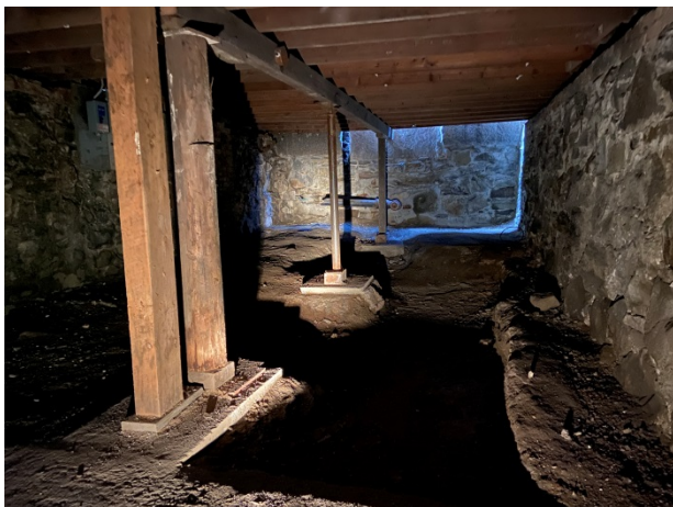
9-Basement looking north
