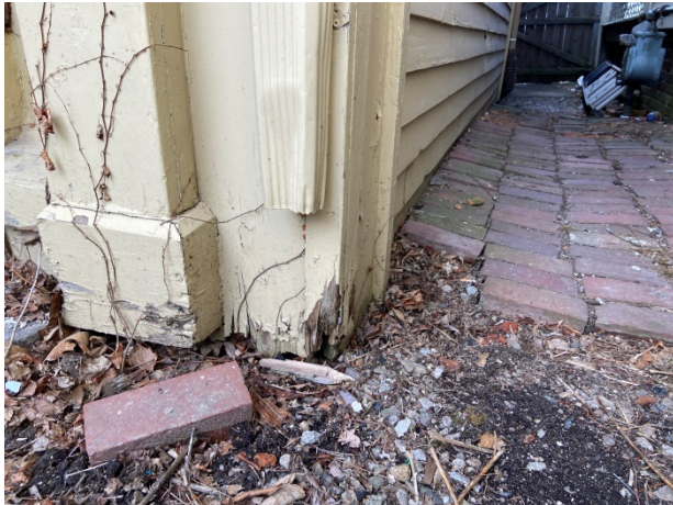
7-Detail at southeast corner
