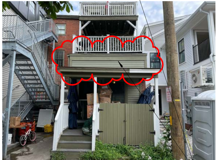
AREA FOR NEW CONDENSERS TO BE WALL MOUNTED 13"-18" ABOVE EXISTING PORCH ROOF
