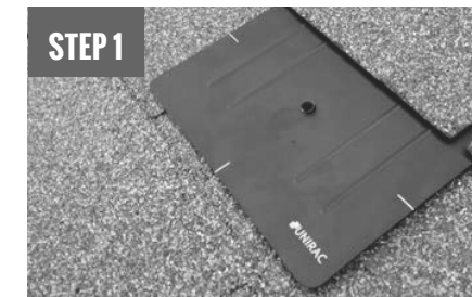
STEP 1 INSTALL FLASHKIT PRO FLASHING
