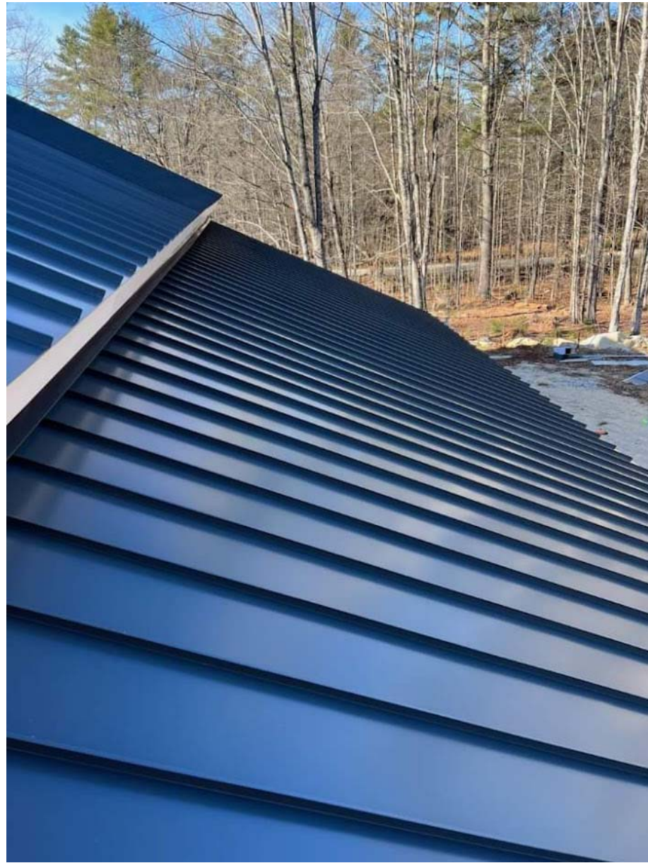
1. STANDING SEAM METAL ROOFING
