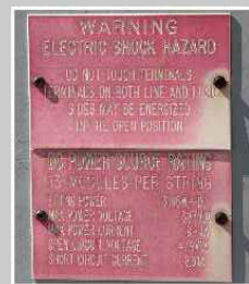
Although placards are generally the most durable option, they need to be designed for exposure
