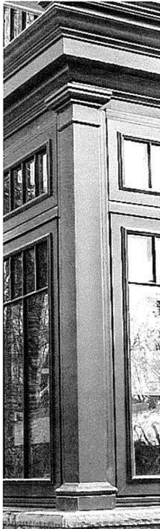
5. CORNER POST COLUMN SURROUND INSULATED ALUMINUM PANEL-BLACK
