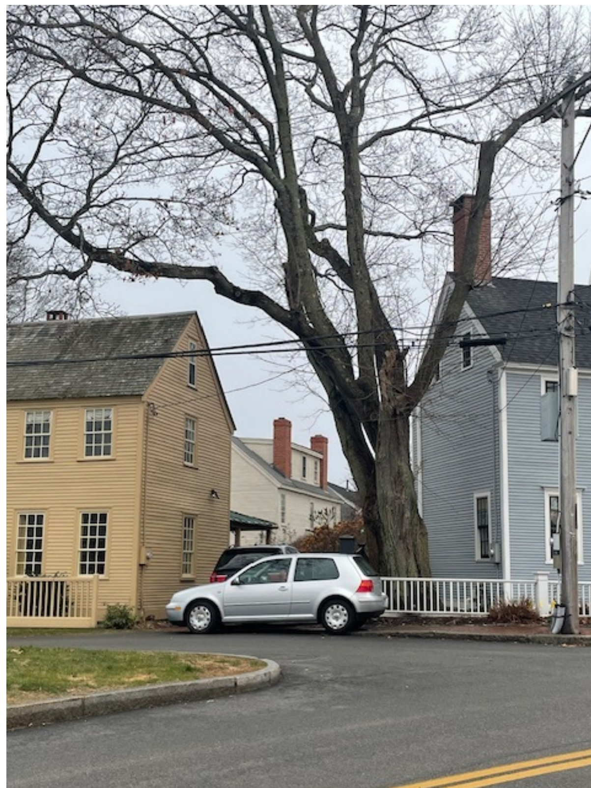
434 MARCY STREET_SHED DORMER STUCK BETWEEN TWO CHIMNEYS
