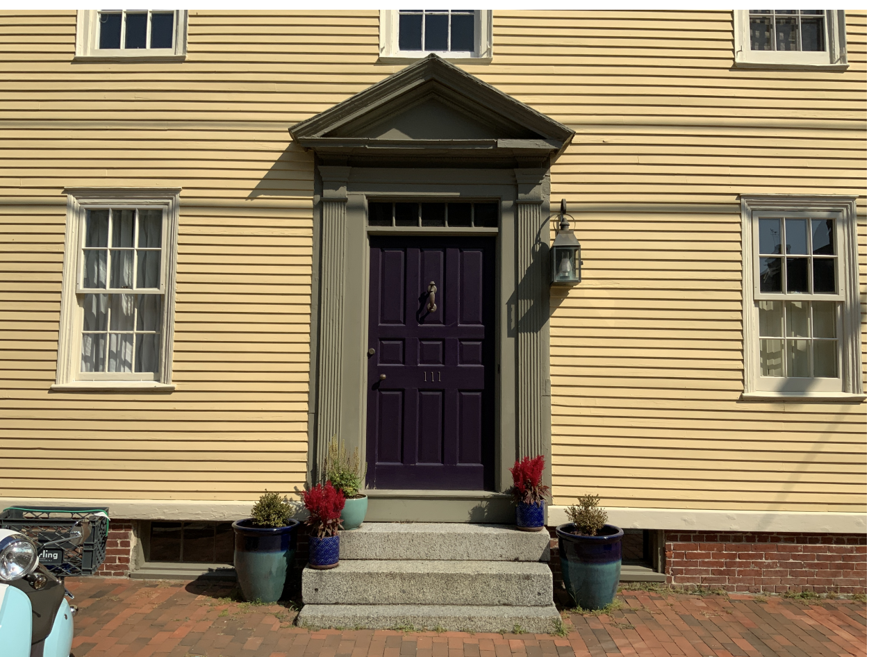
FRONT MAIN DOOR
