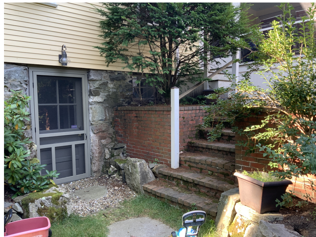
REAR BASEMENT DOOR
