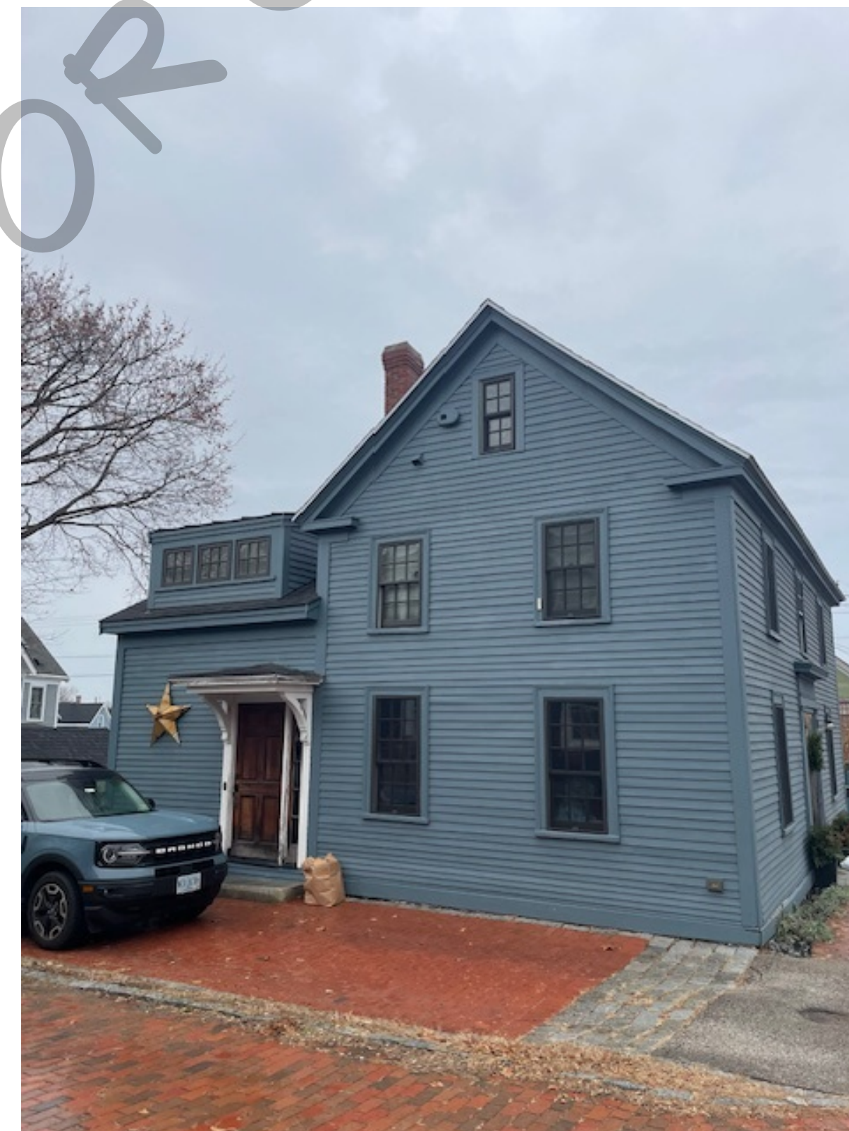
NEW CASTLE AVENUE FRONT SIDE VIEW
