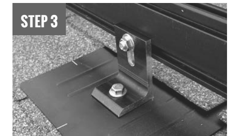
STEP 3 ATTACH L-FOOT TO RAIL
