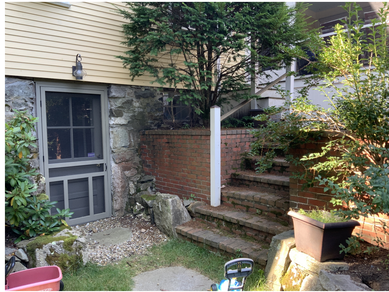
REAR BASEMENT DOOR
