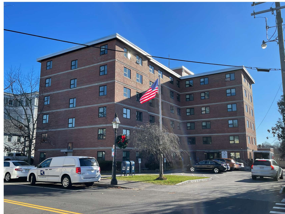
B) VIEW OF EXISTING NORTH & WEST ELEVATIONS
