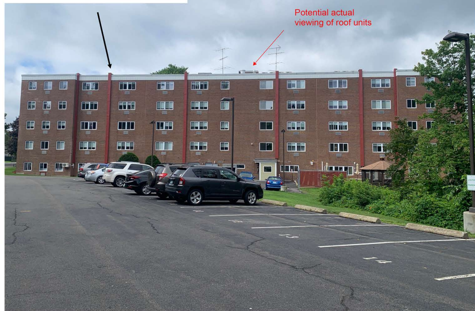
Similar Project—Nutfield Heights, Derry NH Exterior chases shown extending up to roof
