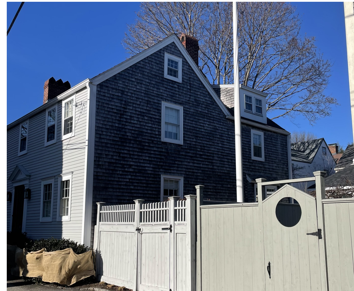
49 HUNKIN STREET_SHED DORMER FACING SIDE
