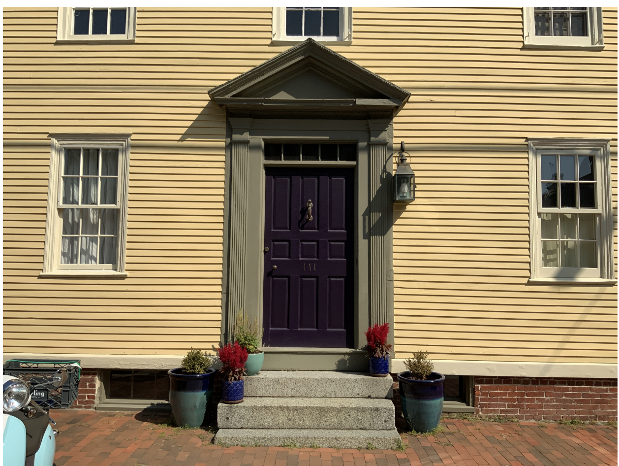
FRONT MAIN DOOR
