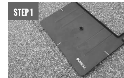
STEP 1 INSTALL FLASHKIT PRO FLASHING
