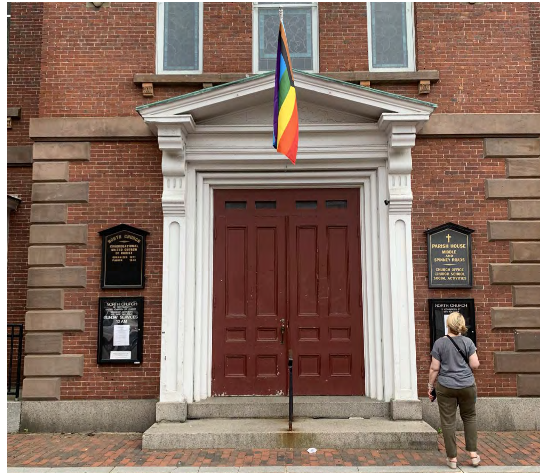
2: EXISTING CENTRAL MAIN ENTRANCE
