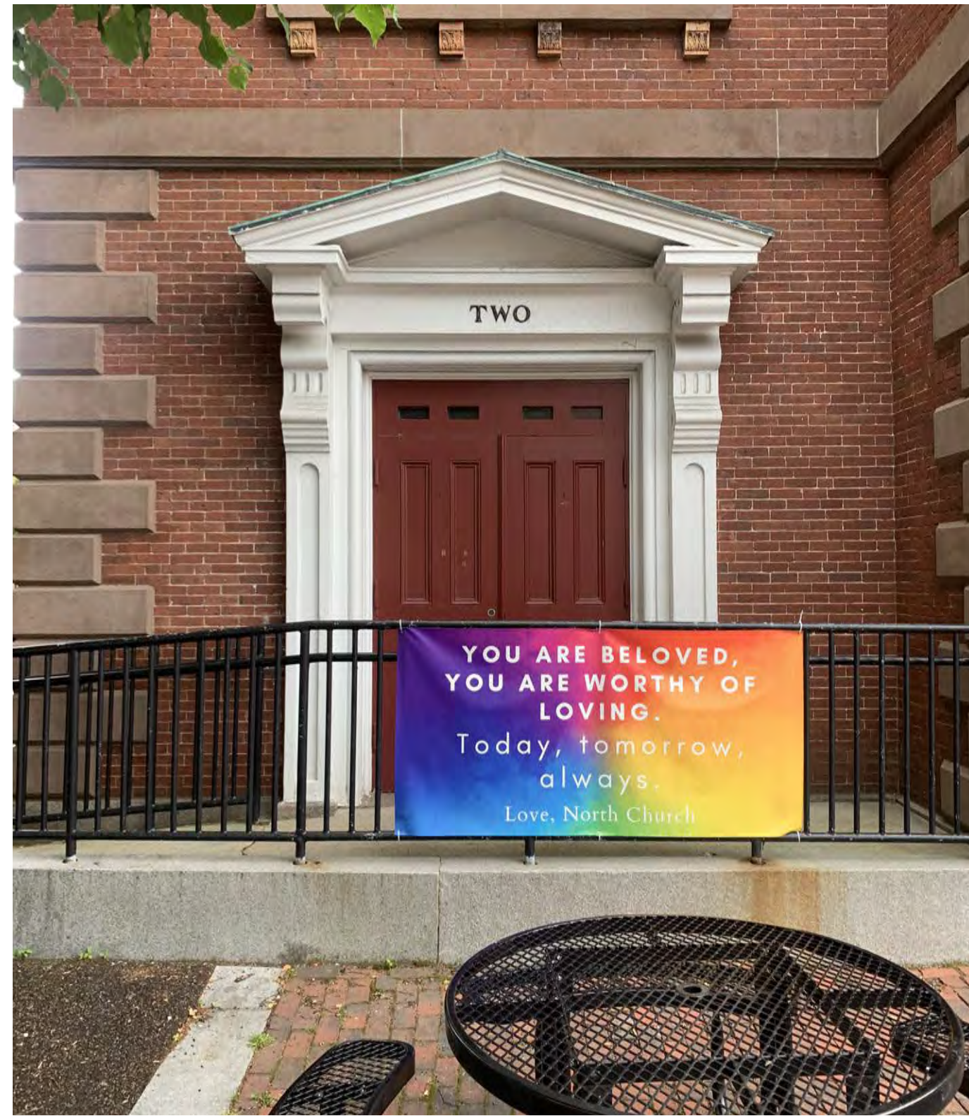
1: EXISTING NORTHEAST ADA ENTRANCE
