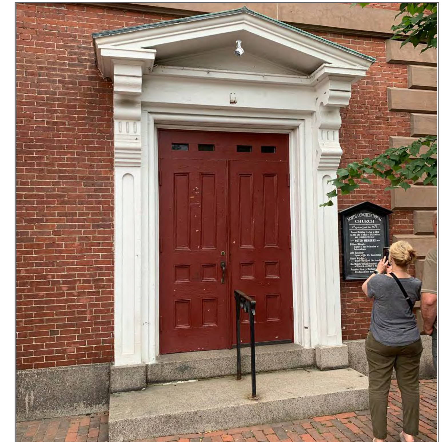
3A: PROPOSED NORTHWEST ENTRANCE New low profile LED spot with minimally invasive installation
