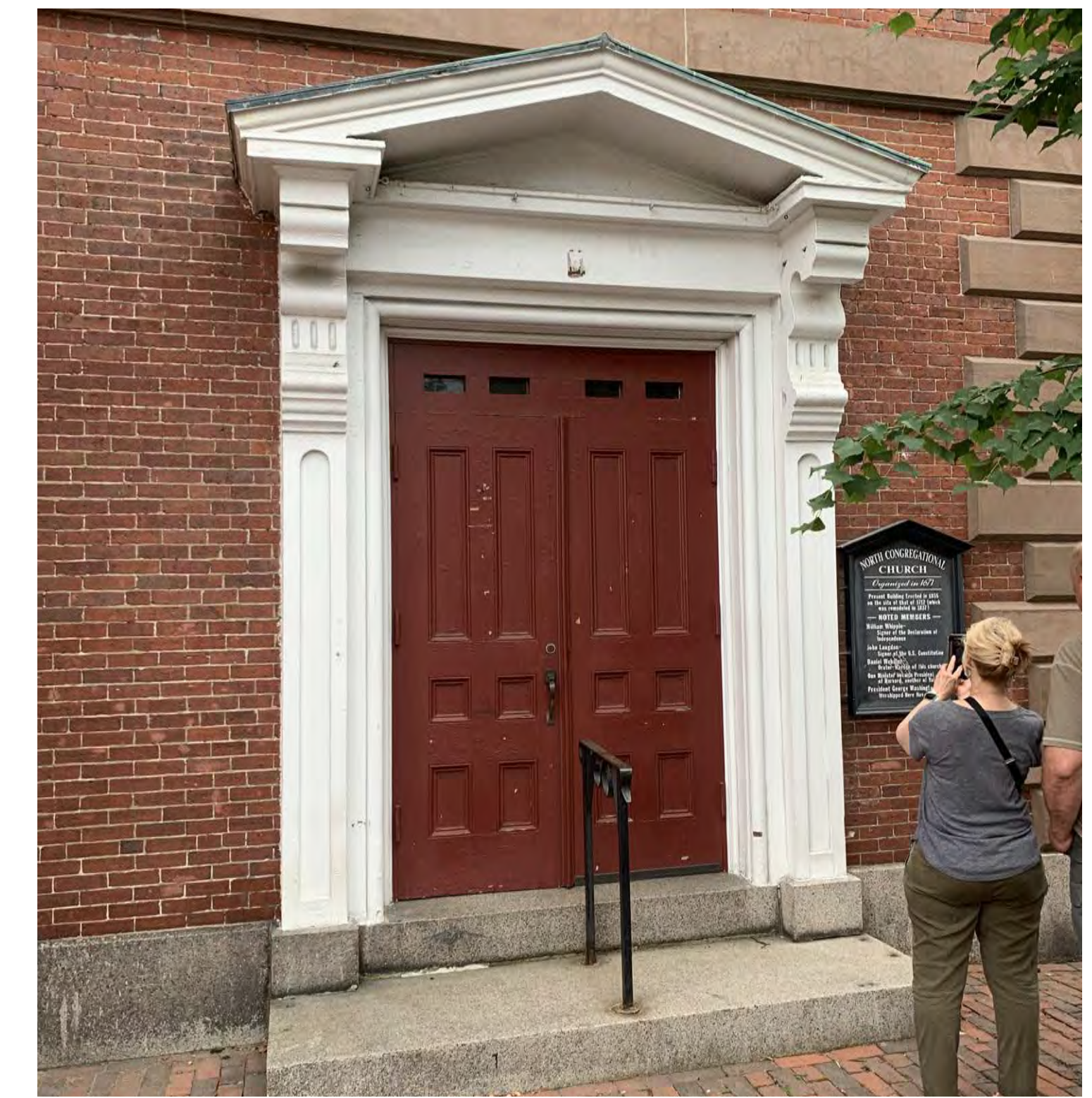
3: EXISTING NORTHWEST ENTRANCE
