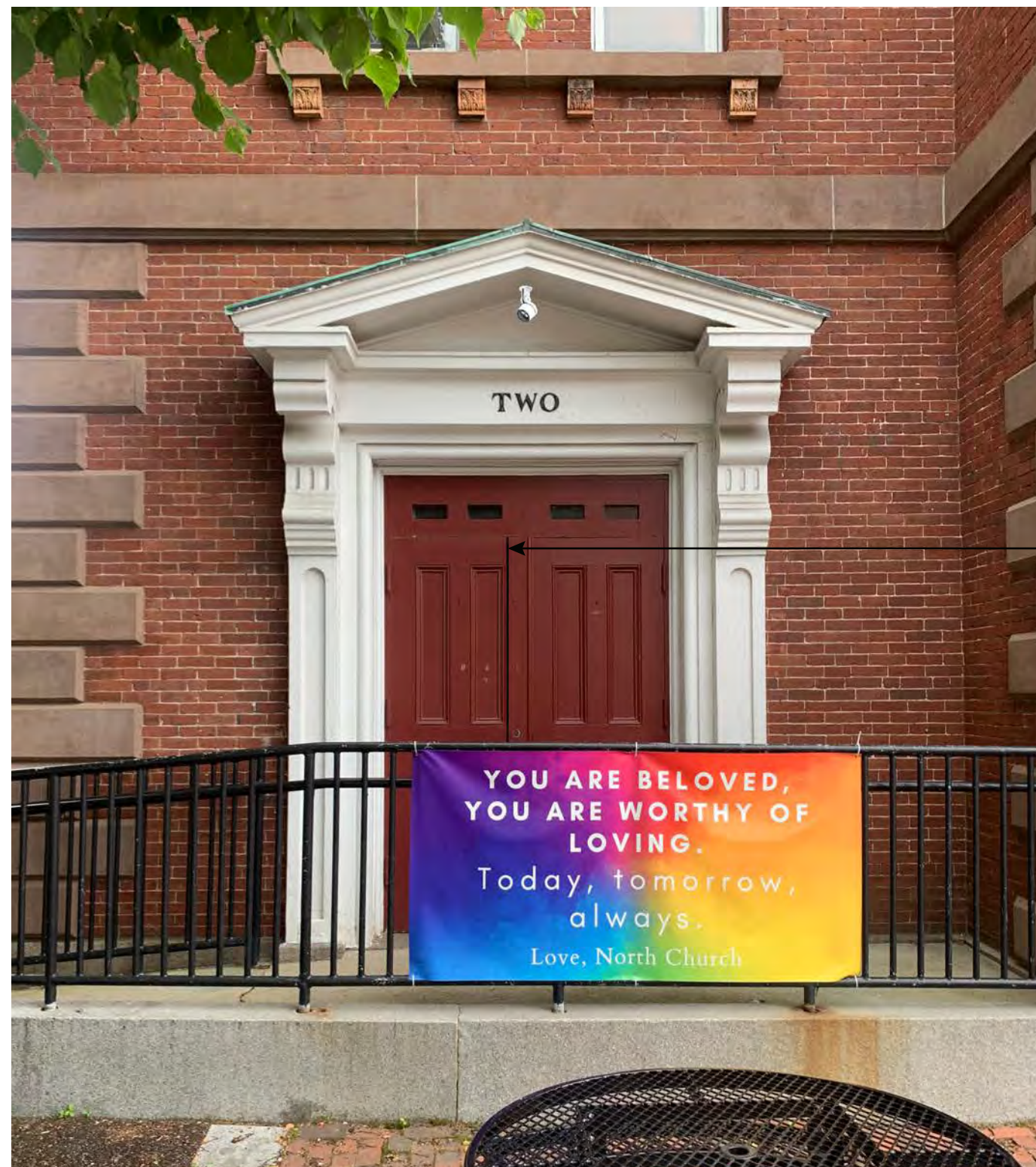
1A: PROPOSED NORTHEAST ADA ENTRANCE New low profile LED spot with minimally invasive installation Door leaf sizes updated to accommodate ADA entry requirements
