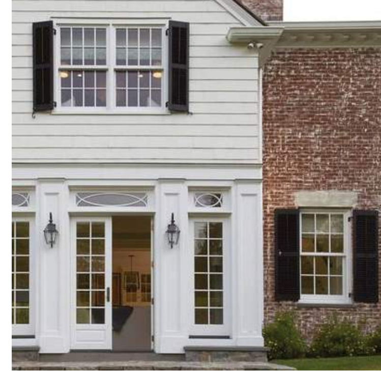
Raised panel with clad and brick
