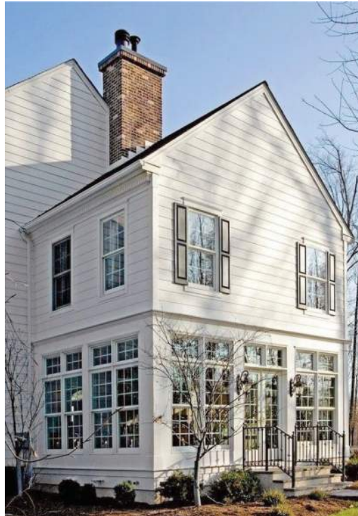
Raised panel wood clad panel above
