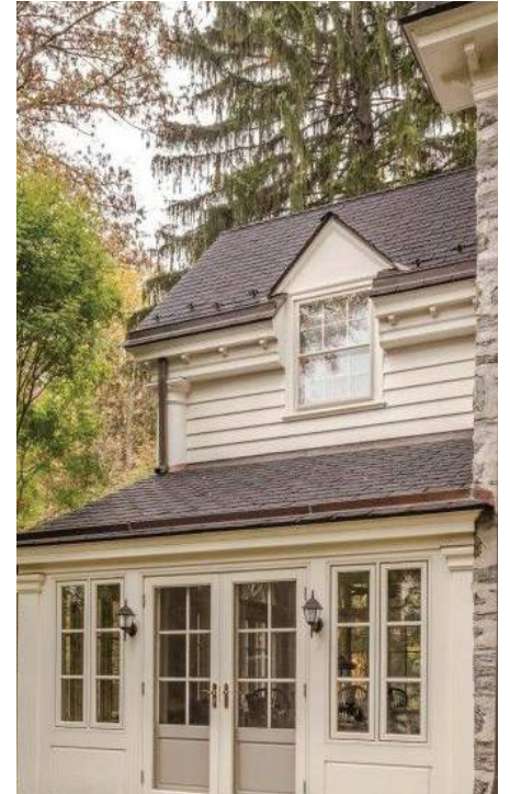
Raised panel with shed above
