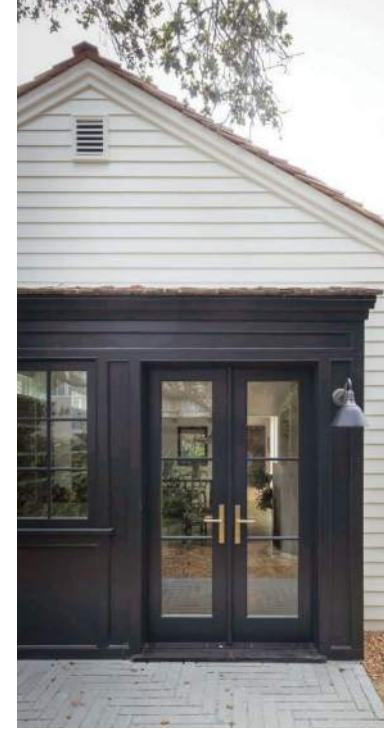
Raised panel with wood clad above
