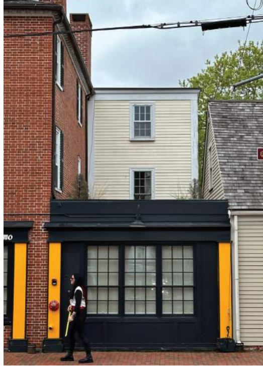
Existing raised panel facade
