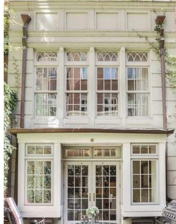
Raised panel facade - Symmetry
