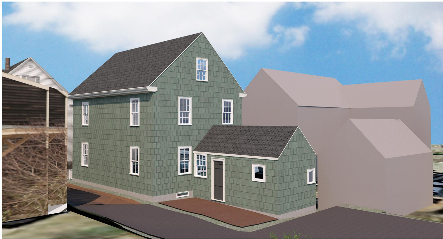
EXISTING SOUTHEAST VIEW
