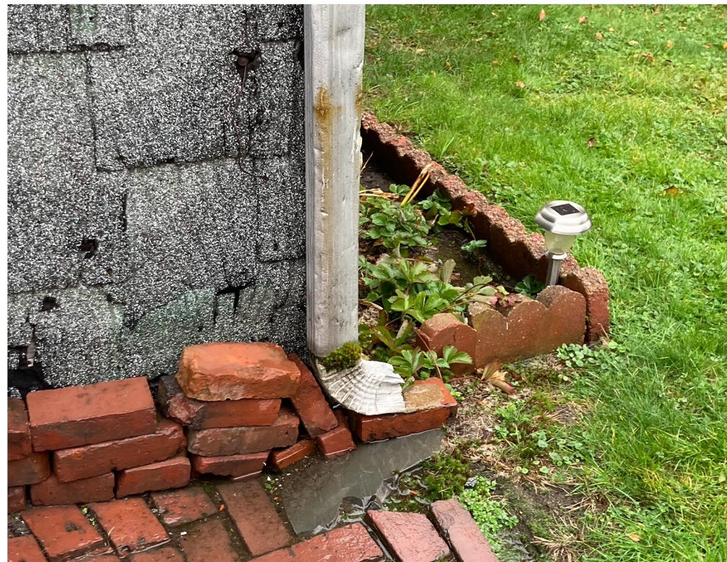
5) VIEW OF EXISTING FOUNDATION AT ATTACHED SHED
