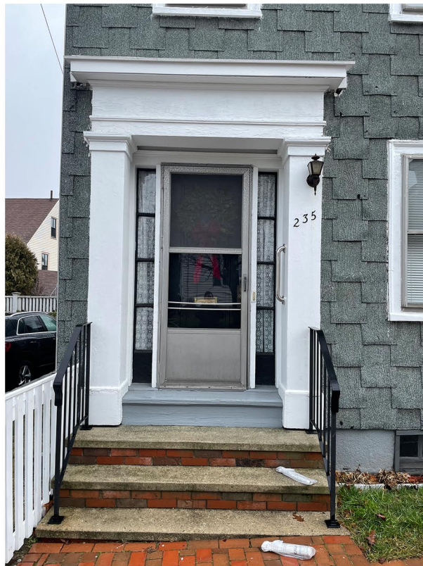
1) VIEW OF EXISTING FRONT ENTRY
