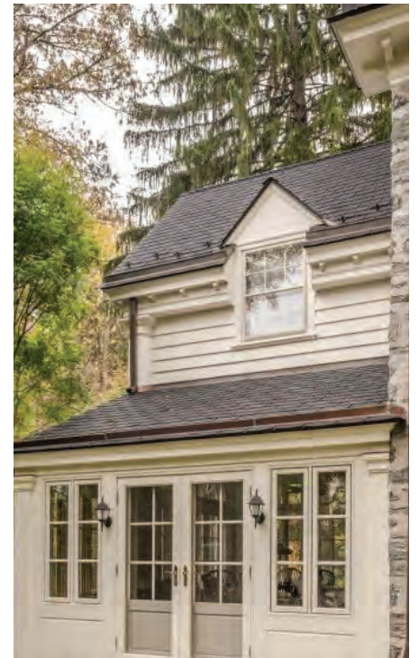
Raised panel with shed above
