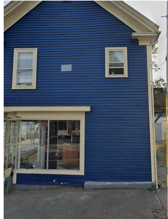
Facade facing Maplewood Ave
