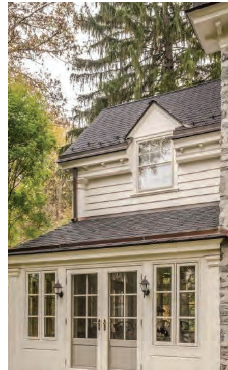
Raised panel with shed above
