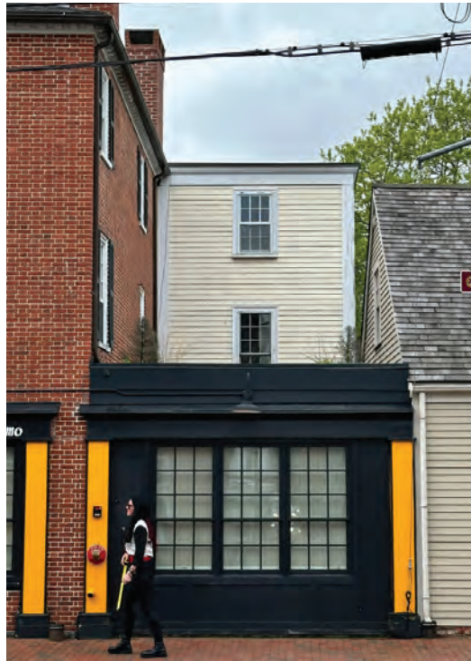
Existing Roof - For slanted across
