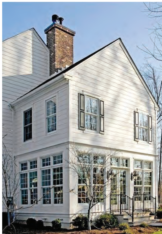
Raised panel wood clad panel above
