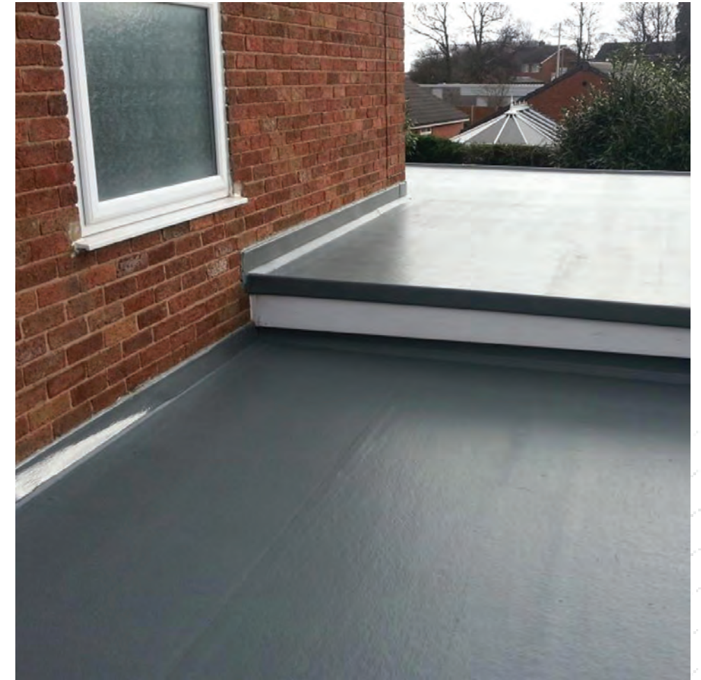
EPDM Rubber membrane roof
