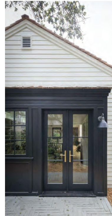
Raised panel with door wood clad above
