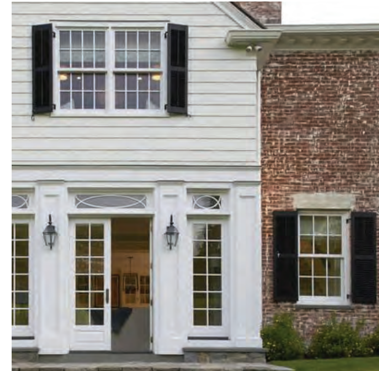
Raised panel with clad and brick
