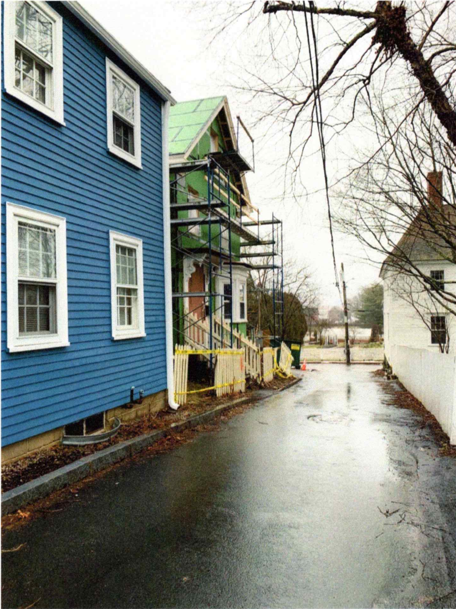
View of Solar Roof from Richmond Street
