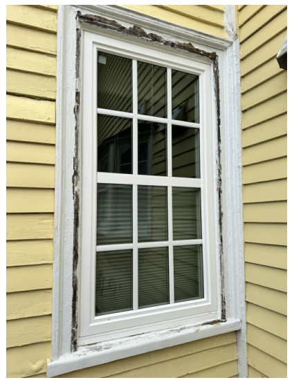
IMAGE WITH REPLACEMENT WINDOWS NOTE: EXISTING DOUBLE HUNG WINDOWS WERE REPLACED WITH CASEMENT WITH A CHECKRAIL FOR CODE COMPLIANCE
