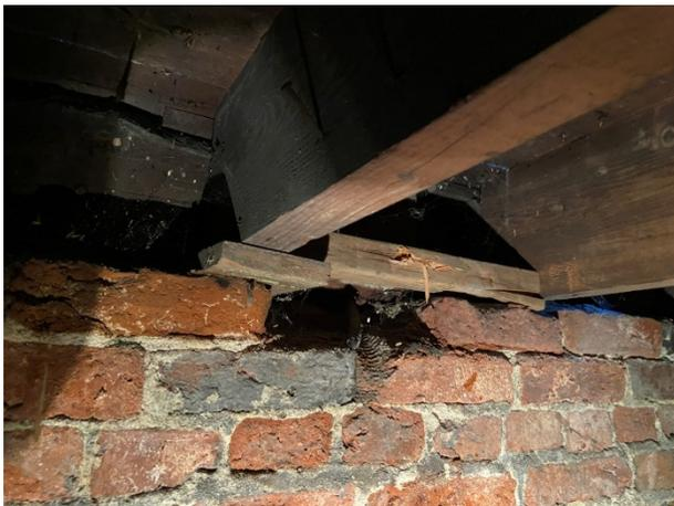
17-Detail of joist end bearing on shims
