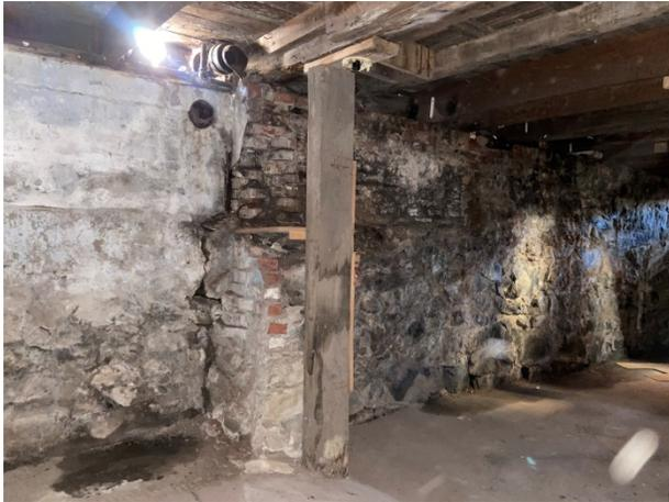
15-Timber post supporting decayed joist
