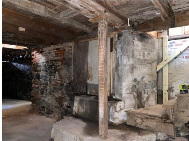
16-Timber post supporting decayed joist
