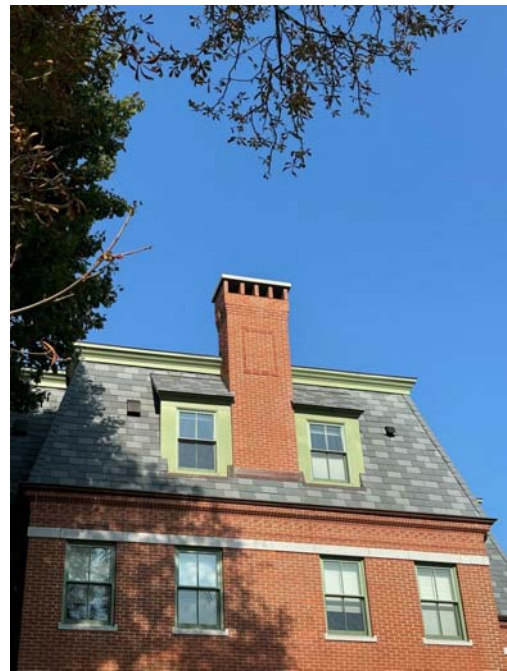
FROM CHAPEL STREET LOOKING NORTH-EAST
