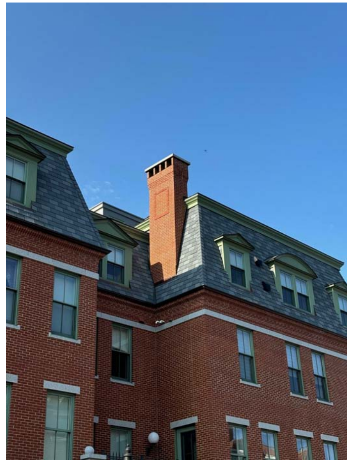
FROM WRIGHT AVE. PARKING LOT LOOKING WEST
