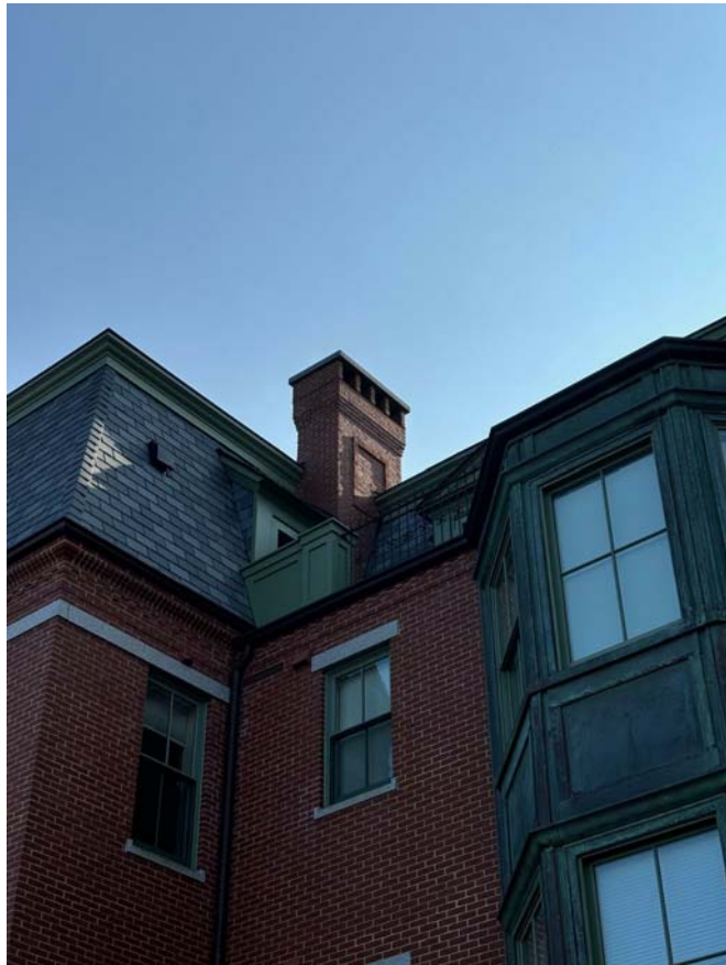
FROM WRIGHT AVE. PARKING LOT LOOKING SOUTH
