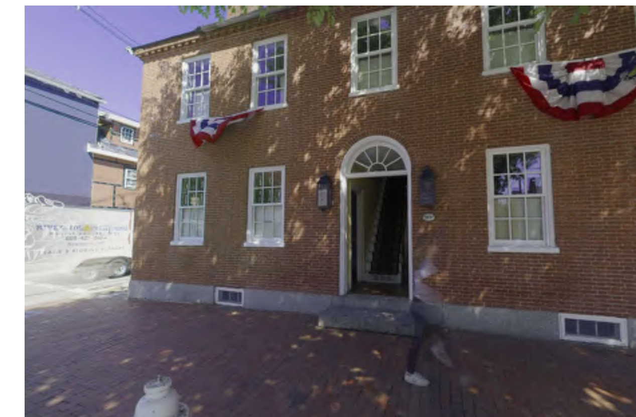
EXISTING STATE STREET ENTRY
