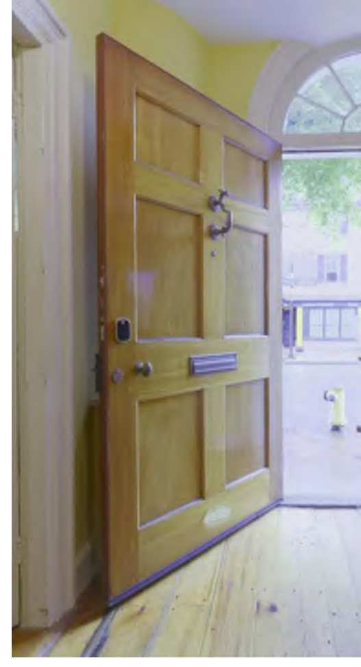
EXISTING STATE STREET DOOR
