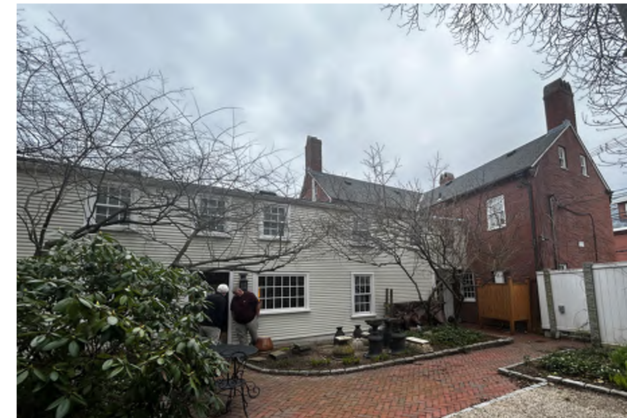
EXISTING REAR CORNER COURTYARD VIEW
