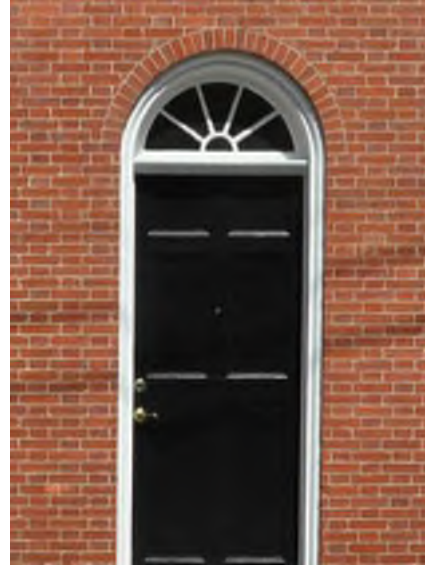
EXISTING DOOR 101 AT CHAPEL STREET
