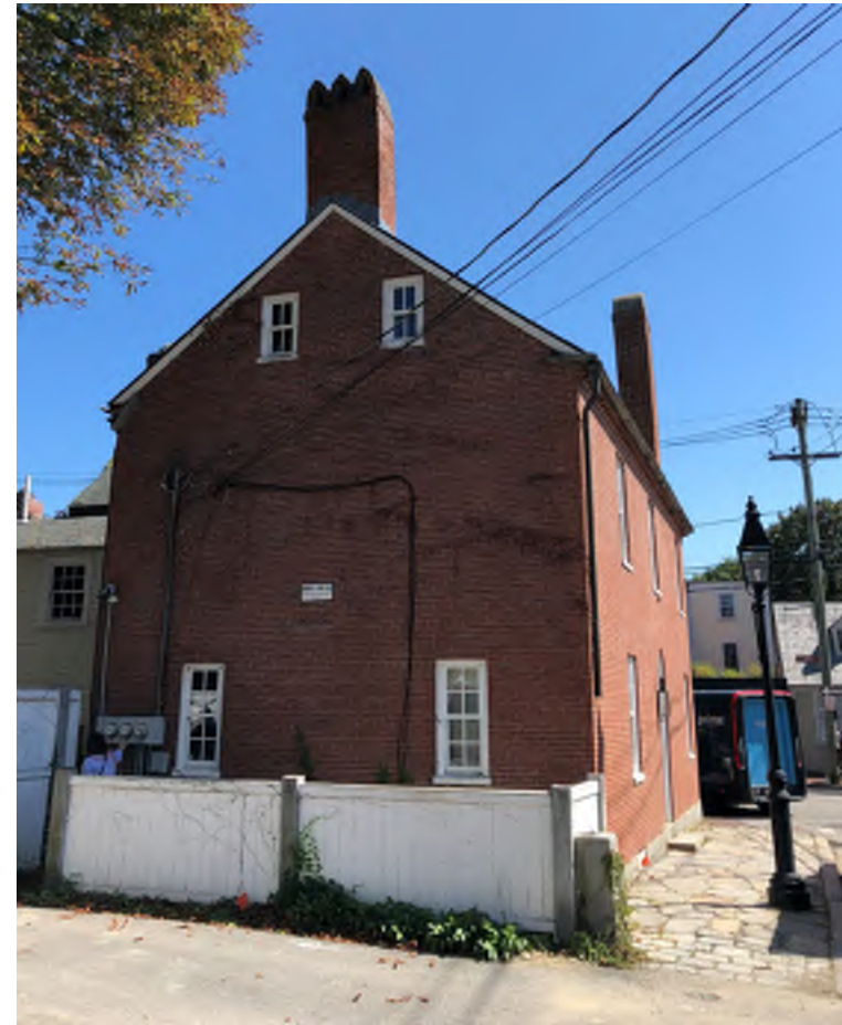
VIEW 1 : VIEW OF FENCED IN MECHANICAL YARD
