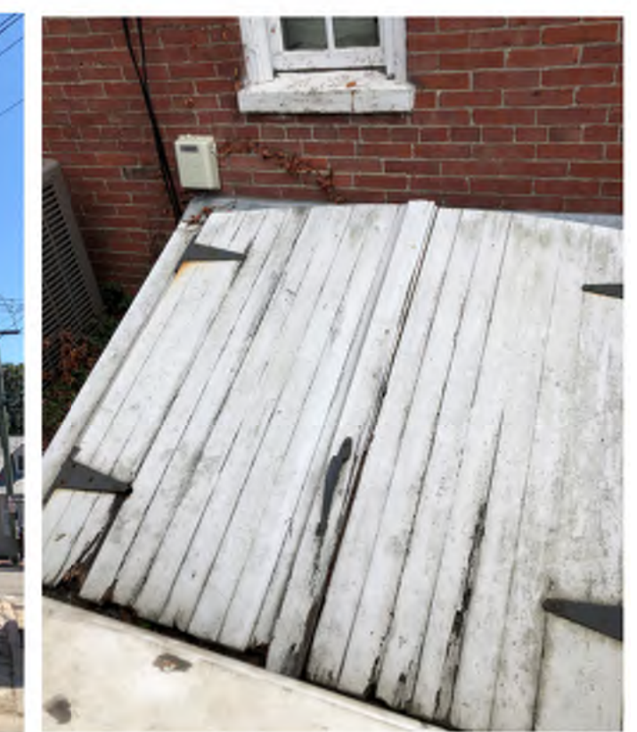
EXISTING BULKHEAD DOOR TO BE REPLACED
