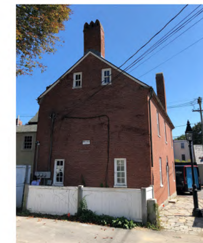
VIEW OF FENCED MECHANICAL YARD
