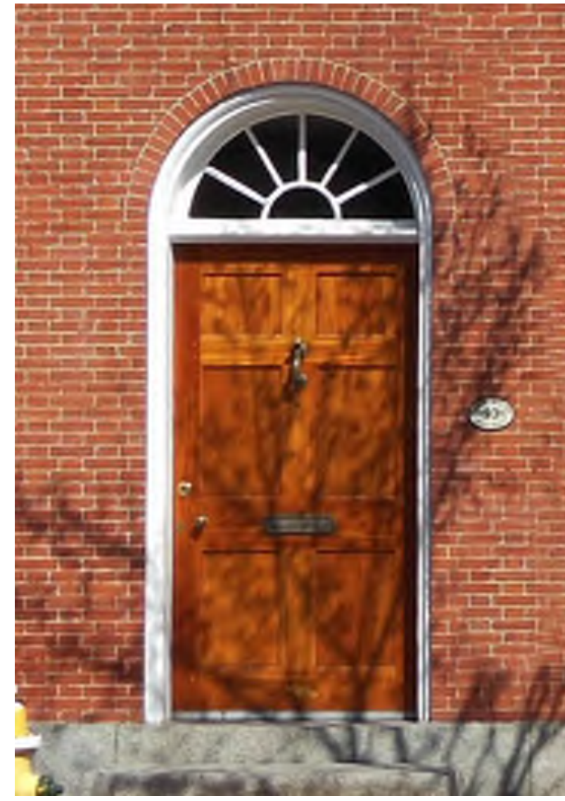
EXISTING DOOR 100 AT CHAPEL STREET
