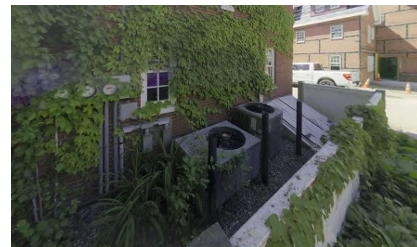
EXISTING MECHANICAL YARD AND BULKHEAD DOOR TO BE REPLACED
