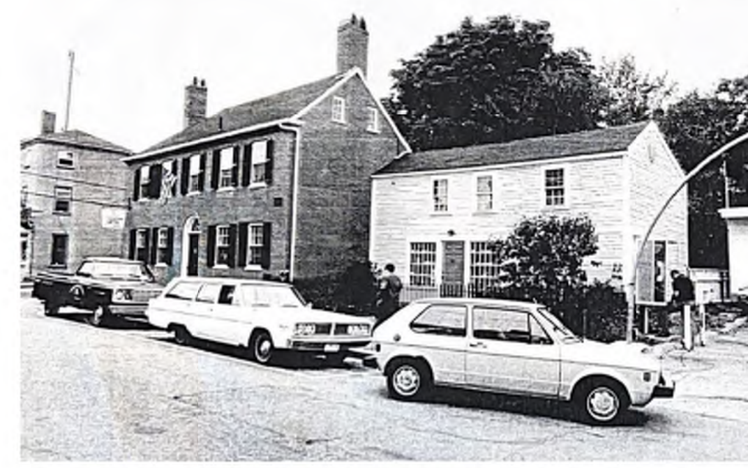
STATE STREET FACADE HISTORICAL PHOTO CIRCA 1970s
