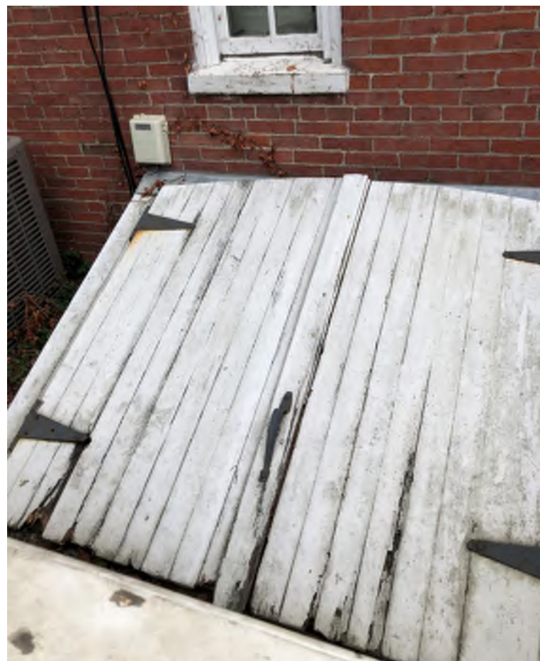
EXISTING BULKHEAD EXTERIOR
