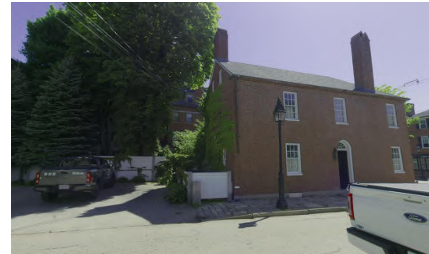
EXISTING CHAPEL STREET VIEW - MECHANICAL YARD BEHIND FENCE
