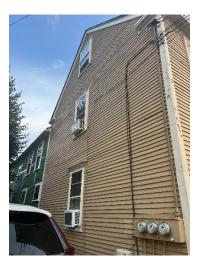
On the south side of the house all 3 windows will be replaced. The 1 window on the lower level will remain nine over six. The 1 window on the second level will remain six over six. The 1 window on the third level will be six over six. See photo below:
