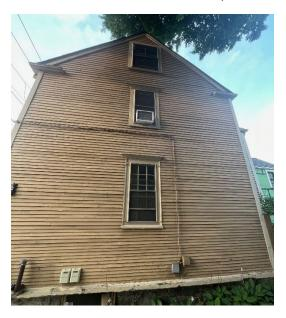
On the west side (the back corner of the house) all 3 windows will be replaced. The 1 window on the lower level on the left will remain nine over six. The 1 window on the lower level on the right will remain six over six. The second level window will remain six over six. See photo below:
