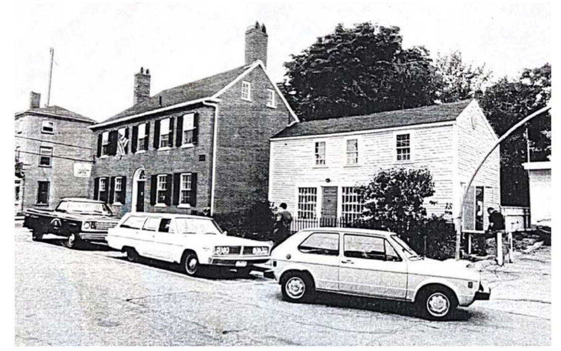
STATE STREET FACADE HISTORICAL PHOTO CIRCA 1970s
