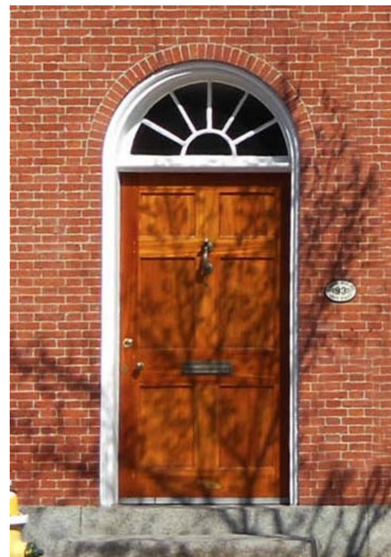
EXISTING DOOR 100 AT CHAPEL STREET
