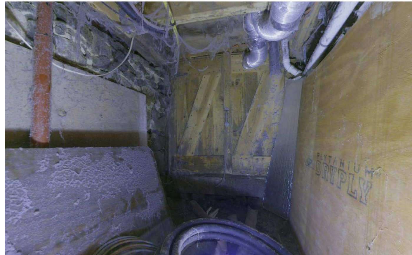
VIEW 1 : VIEW OF EXISTING BULKHEAD FROM INTERIOR
