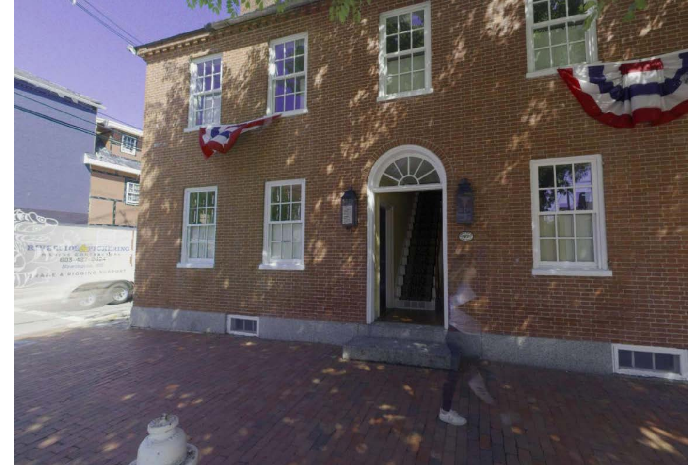
EXISTING STATE STREET ENTRY
