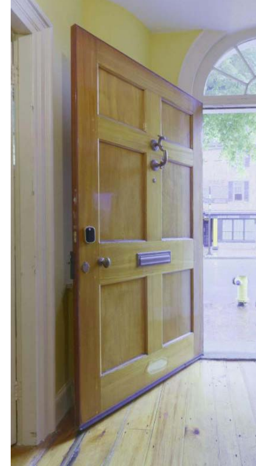
EXISTING STATE STREET DOOR
