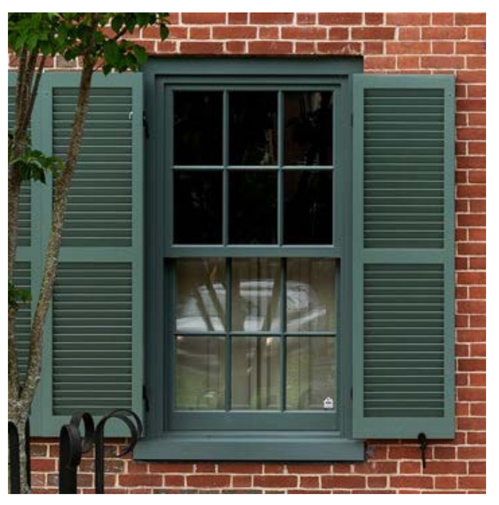
EXAMPLE IMAGE OF LEPAGE SIMULATED DIVIDED LITE W/ SPACER BAR WINDOW WITH SHUTTERS 129 DANIEL STREET, PORTSMOUTH, NH
