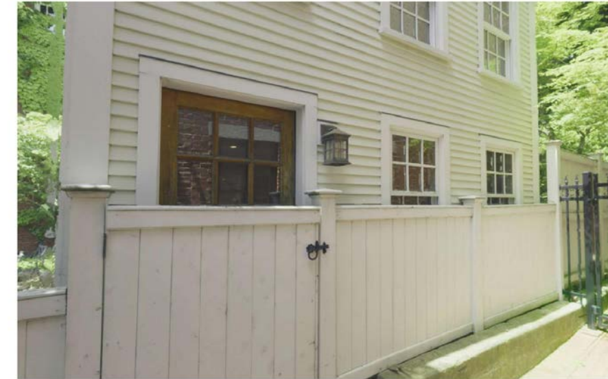
EXISTING ALLEYWAY FENCE OBSTRUCTING WINDOWS & DOORS
