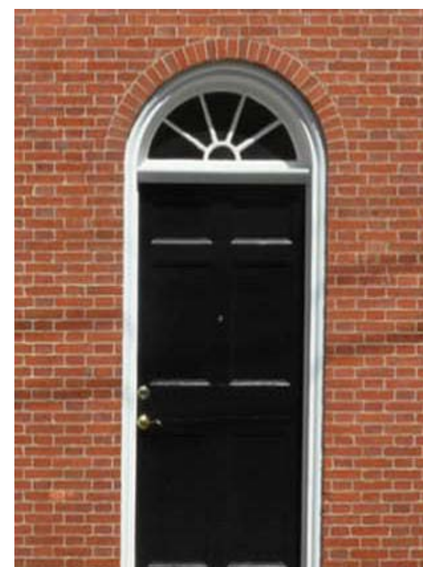
EXISTING DOOR 101 AT CHAPEL STREET
