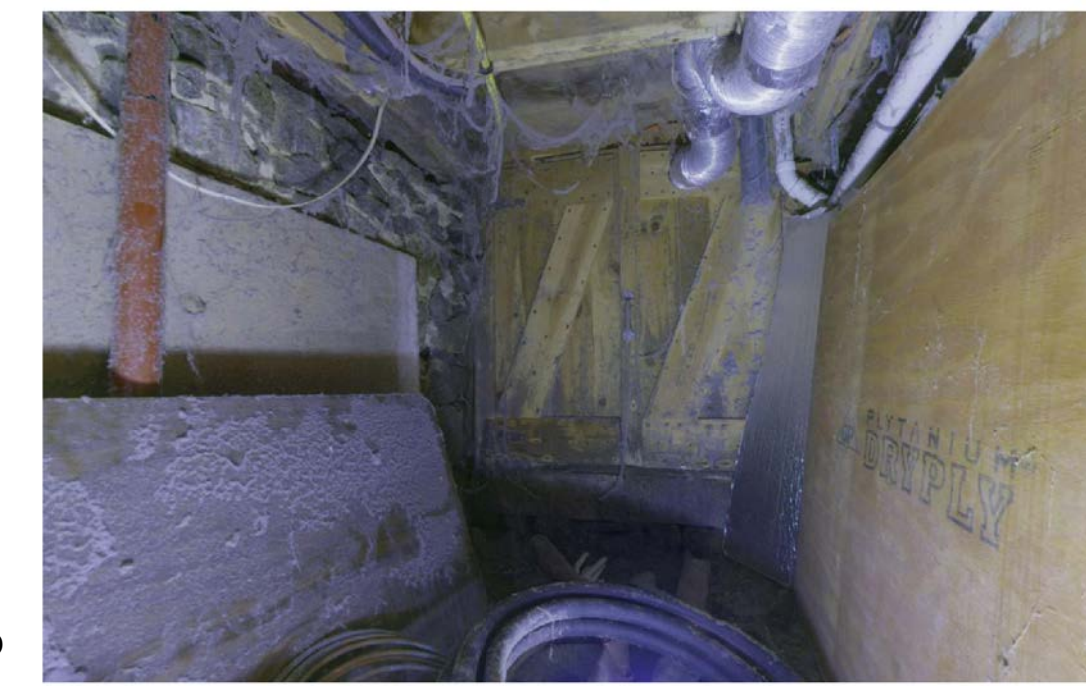
EXISTING BULKHEAD INTERIOR
