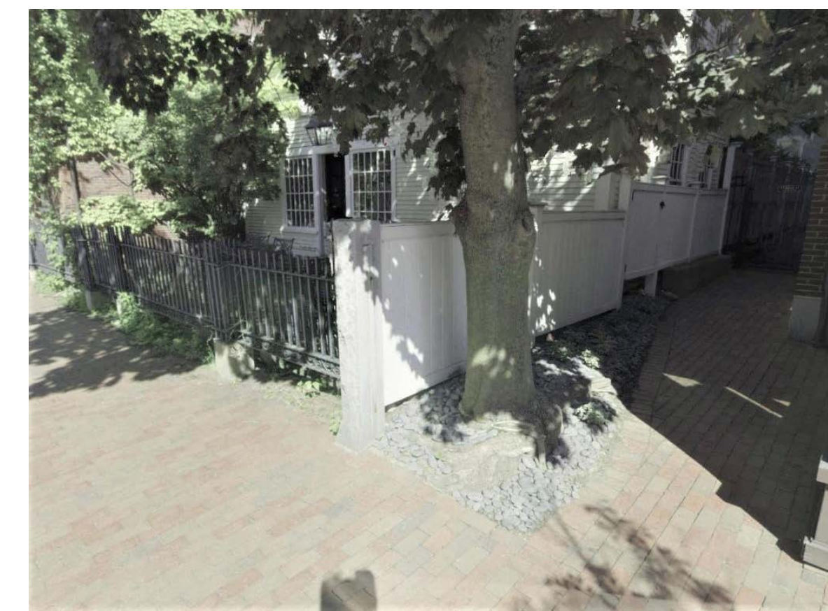
EXISTING STATE STREET ALLEYWAY TREE AND FENCE
