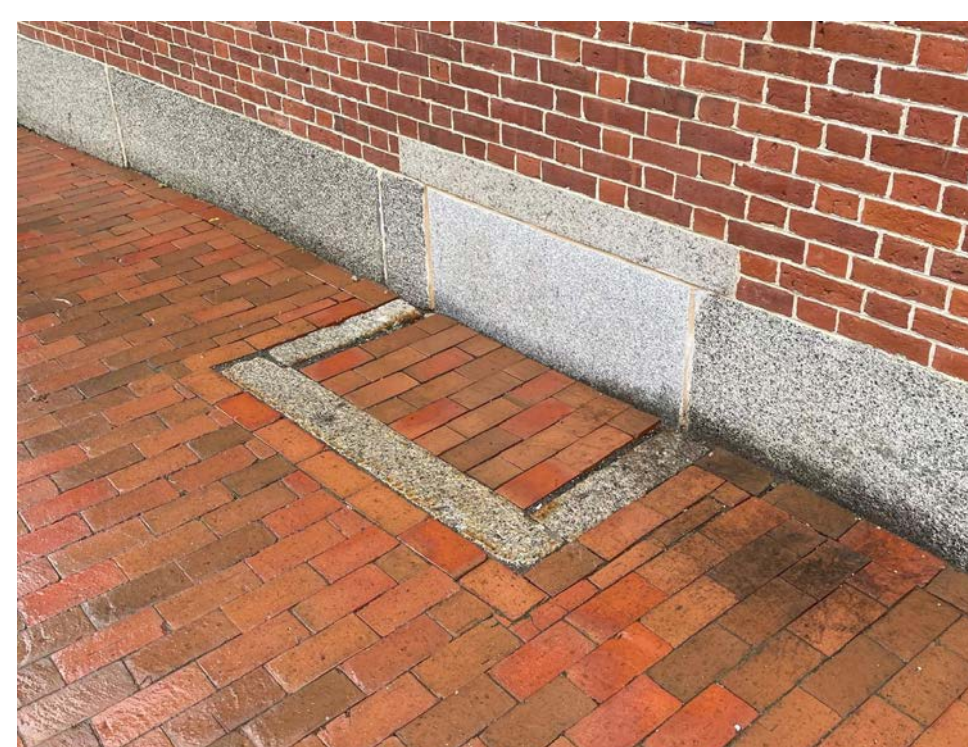
PROPOSED STONE INFILL EXAMPLE **FOR REFERENCE ONLY** DESIGN INTENT TO MATCH EXISTING STONE.
