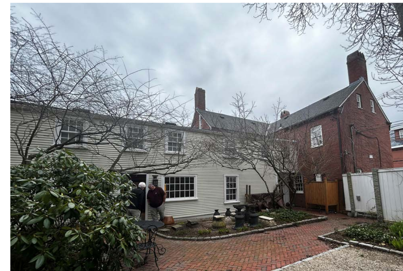
EXISTING REAR CORNER COURTYARD VIEW
