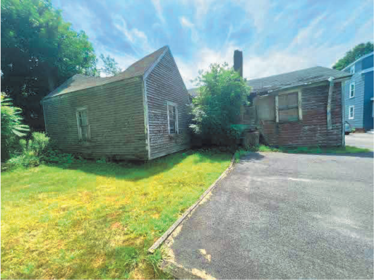
Accessory Building (Rear View)
