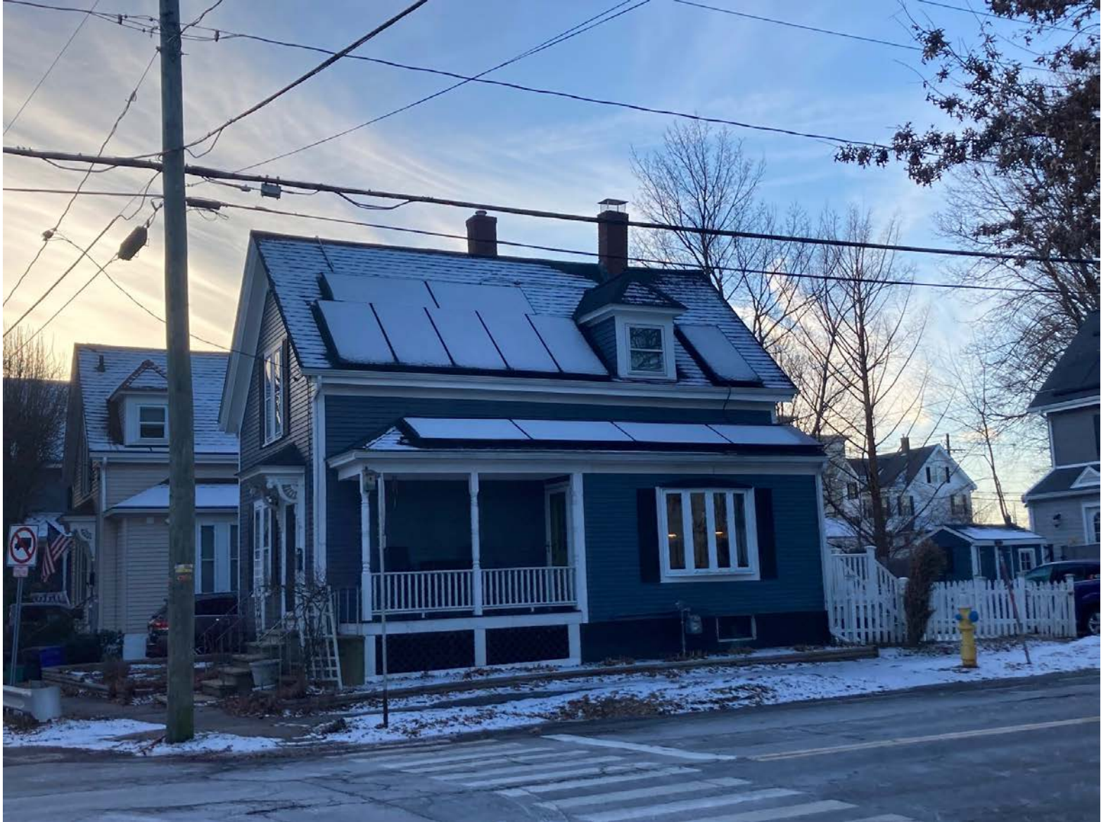
Bartlett and Thornton Streets-Visible 14
