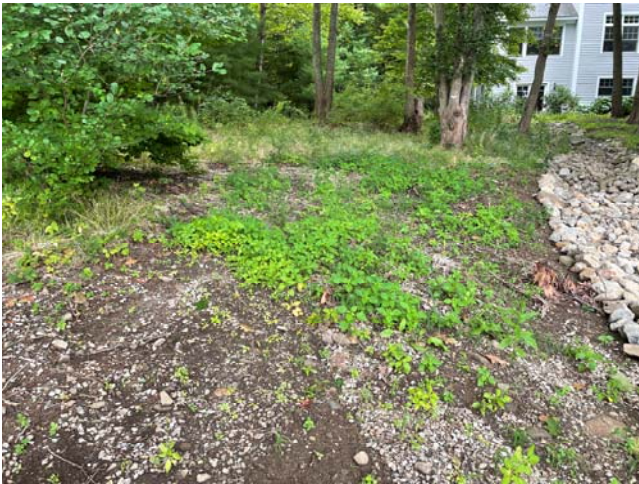
Figure 1. Downstream end of swale and discharge by improved stone wall end (top left); stone swale looking upstream, photo taken from area close to stone wall end (right); property directly north of swale subject to erosion, looking upstream, photo taken from area close to stone wall end (lower left).
