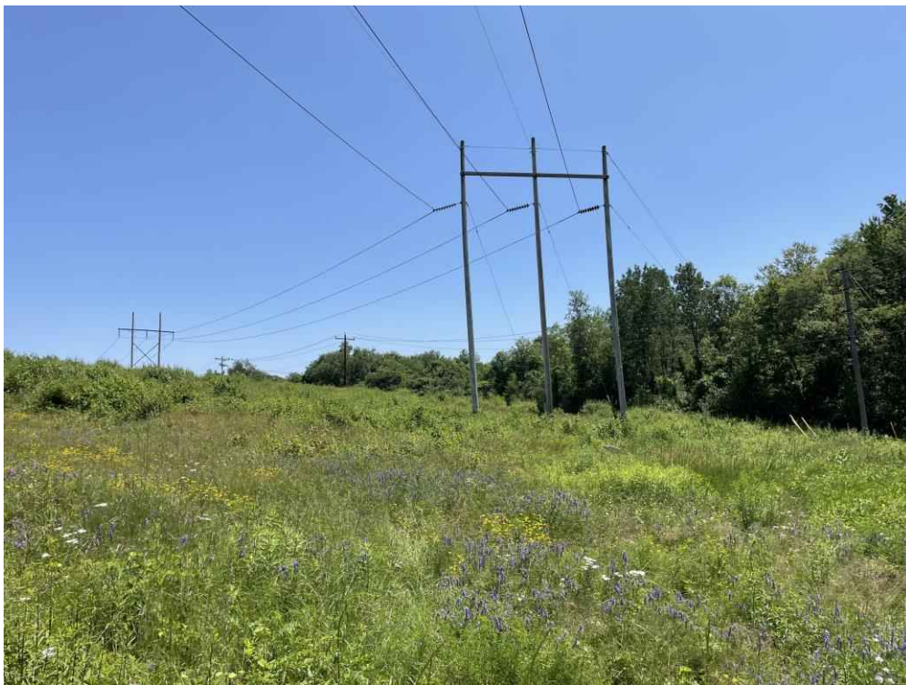
Photograph No. 28: Looking southeast at Structure 4 on the T13 Line ROW off Gosling Road, Portsmouth, NH.
