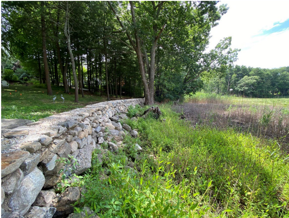
Photo 8. Overview of the downslope side of the stone wall, viewing south from the northern end of the stone wall. Wetland POGW1 occurs in the right side of the photo. (08-11-22)
