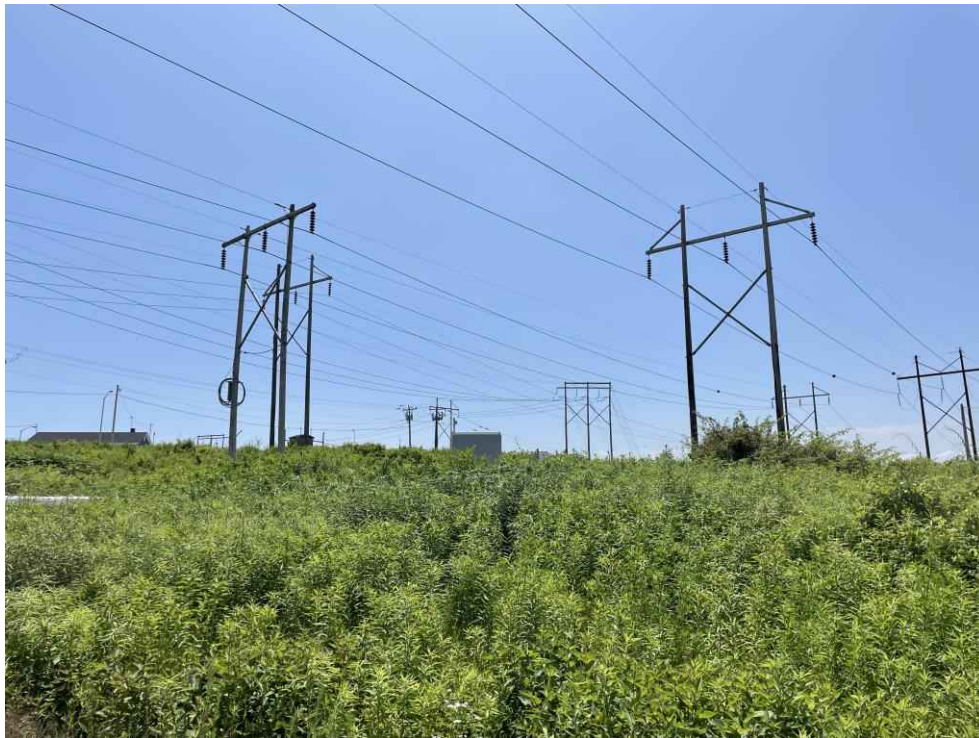
Photograph No. 22: Looking south near Wetland PW-2 (PEM1/PSS1E) on the T13 Line ROW off Gosling Road, Portsmouth, NH.
