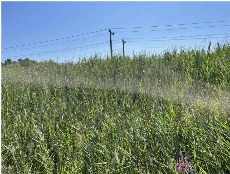
Photograph No. 4: Looking east at Wetland GW-1 (PEM1/PSS1/PFO1E.Fg/R2UB) near Structure 92 on the 3171 Line ROW off Ocean Road, Portsmouth, NH.
