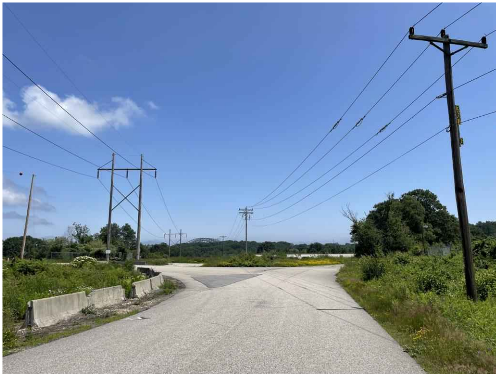
Photograph No. 32: Looking east at Structure 7 and Wetlands PW-10 (PSS1Ex) and PW-11 (PSS1/PEM1Ex) on the T13 Line ROW off Gosling Road, Portsmouth, NH.
