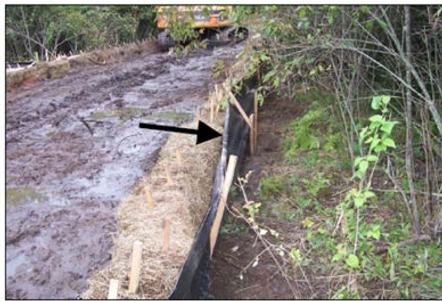
Properly installed hay bale barrier with silt fence (direction of flow indicated by arrow).
