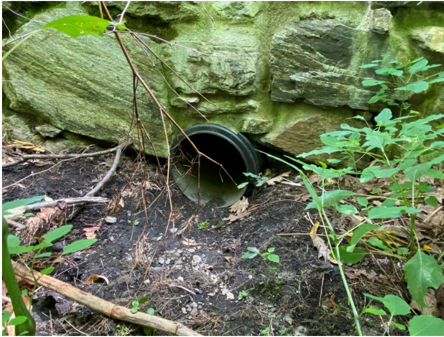
Southern culvert outflow serving as the delineated upstream end of POGS1 in wetland POGW2. (08-11-22)
