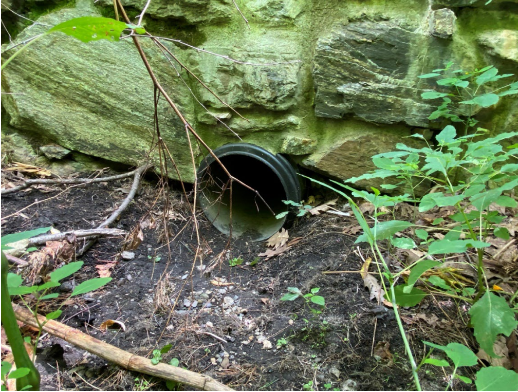
Photo 17. Southern culvert outflow (source of POGS1) into POGW2, viewing west. (08-11-22)
