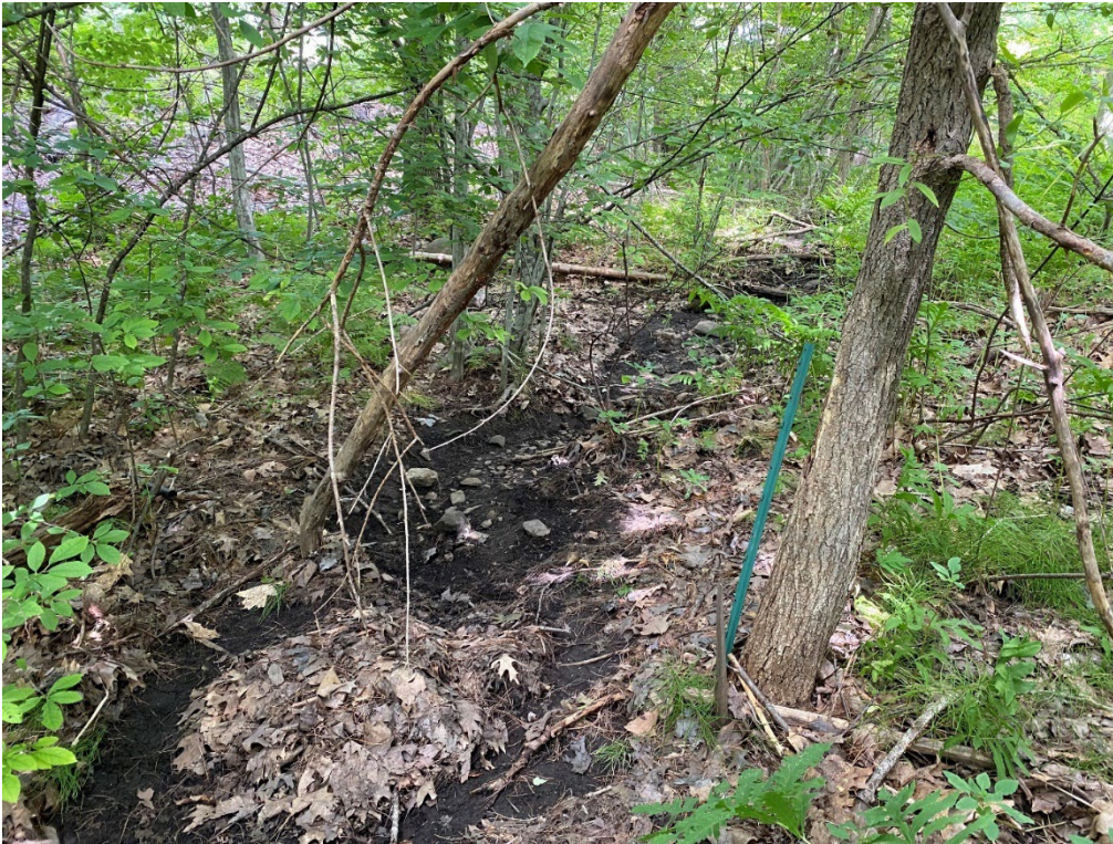
Photo 21. POGS1 leading onto the Gardner property from the culverts located at the northeastern end of POGW2, viewing southwest, downstream. Property boundary is indicated by the green rod visible in the right side of the photo. (08-11-22)
