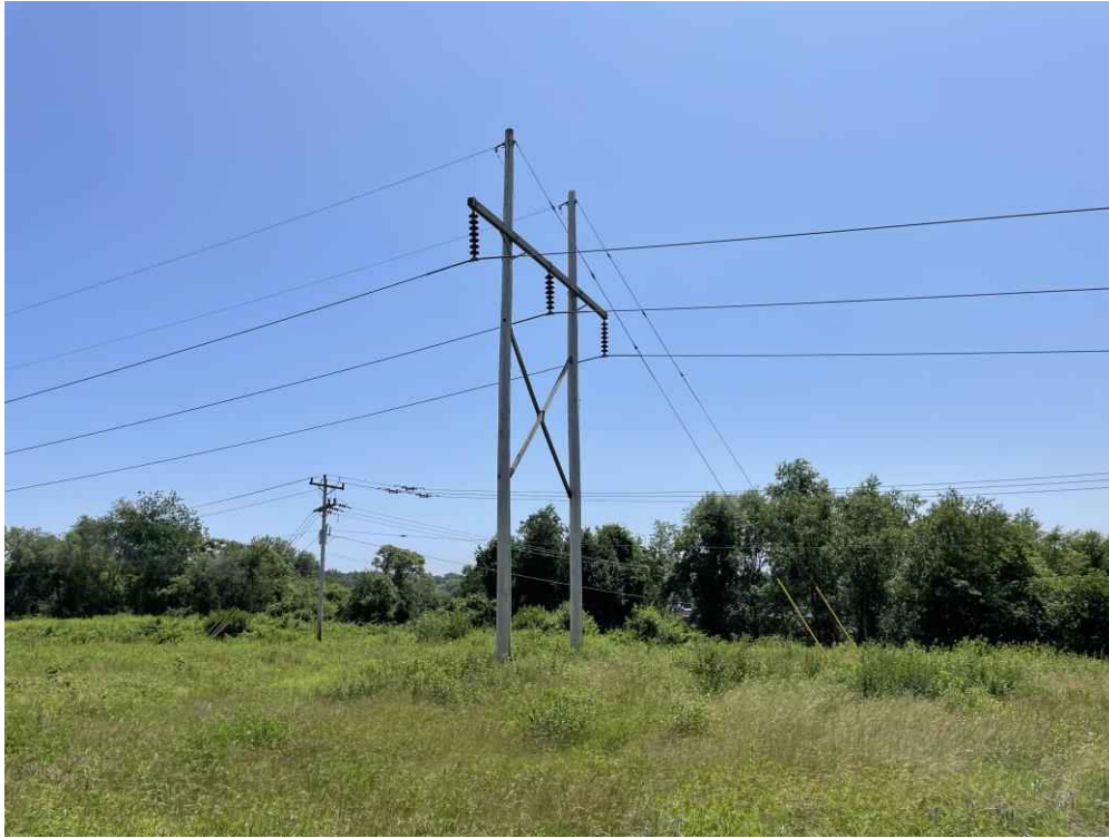
Photograph No. 29: Looking south at Structure 5 on the T13 Line ROW off Gosling Road, Portsmouth, NH.
