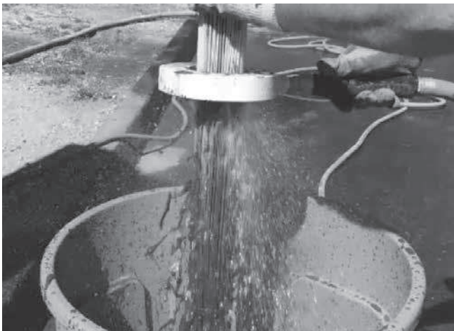
Vacuuming Sump Through MAW
