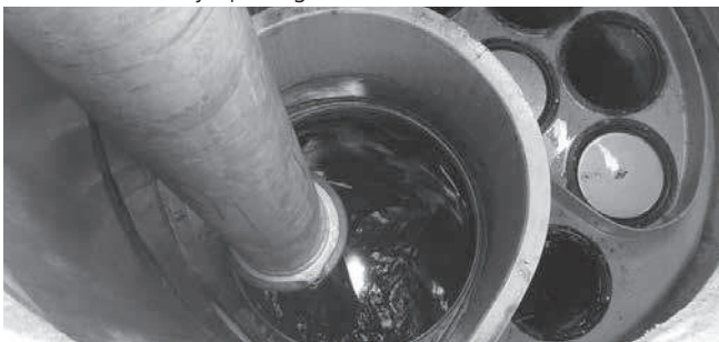
Vacuuming Sump Through MAW
