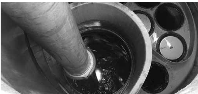
Vacuuming Sump Through MAW
