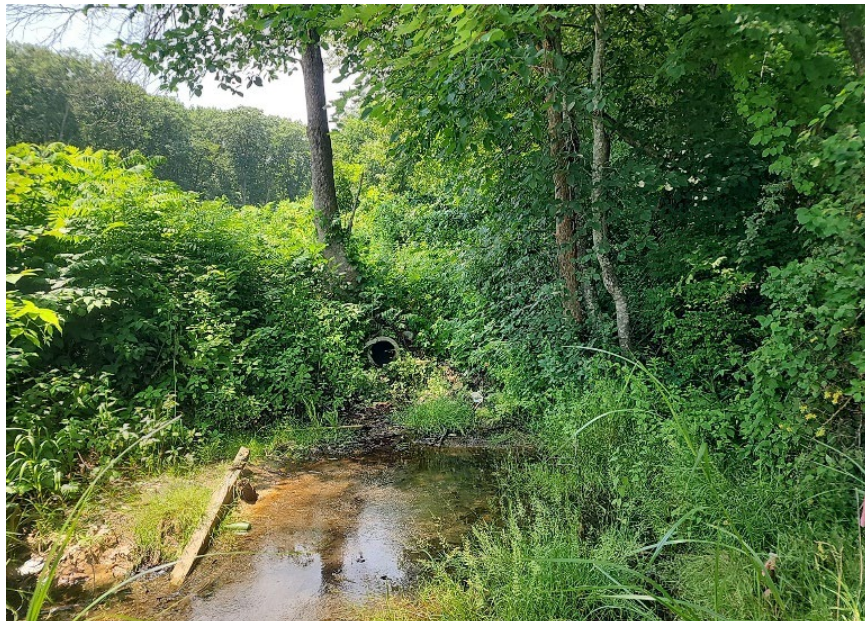
Photograph 8b: Looking north, storm drain pipe underneath green ash tree, pipe above highest observable tide line; July 2024
