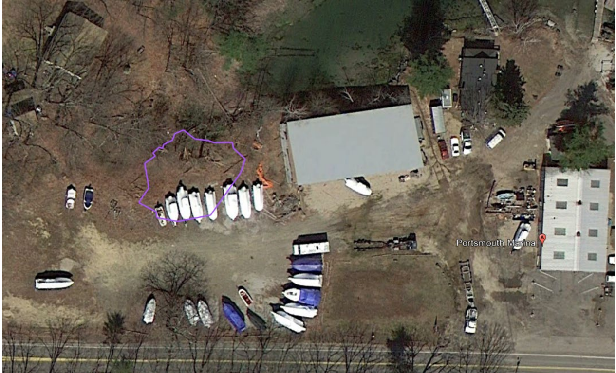
Photo 2: April 2013 Google Earth Image – Approximate 2016-2017 PCB excavation extents outlined in purple.
