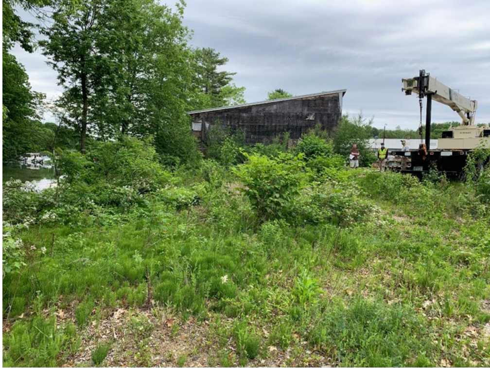
Photo 6: June 2020 - Witch Cove on left, PCB excavation area (overgrown) in foreground. Former marina building in background. View to east.
