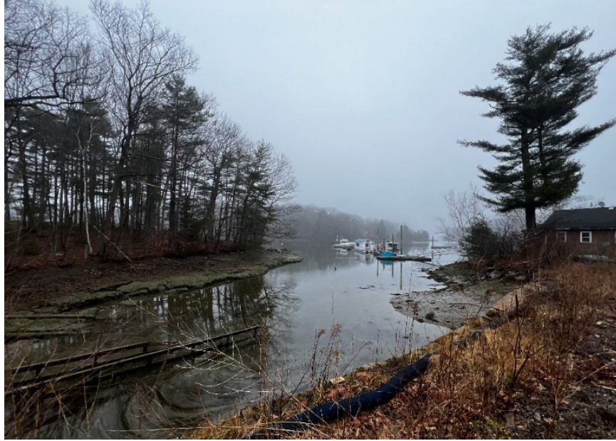
Photograph 4a: Looking east, east of wetland remediation area and berm, in vicinity of cribbed retaining wall and building foundation, at right; April 2024
