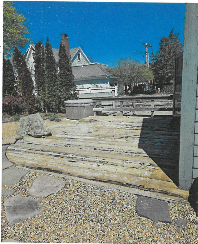
Photo #17: Looking northwesterly at existing deck to be replaced. April 28, 2025
