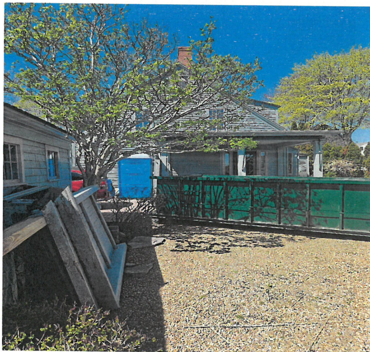
Photo #14: Looking westerly towards the covered deck to be modified into a sun porch with deck above. April 28, 2025
