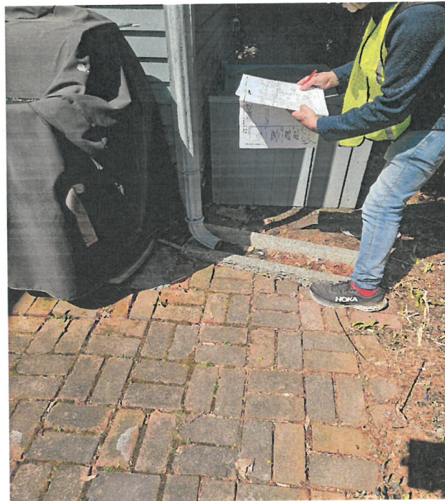
Photo #20: Looking southwesterly at existing downspout and HVAC system. April 28, 2025
