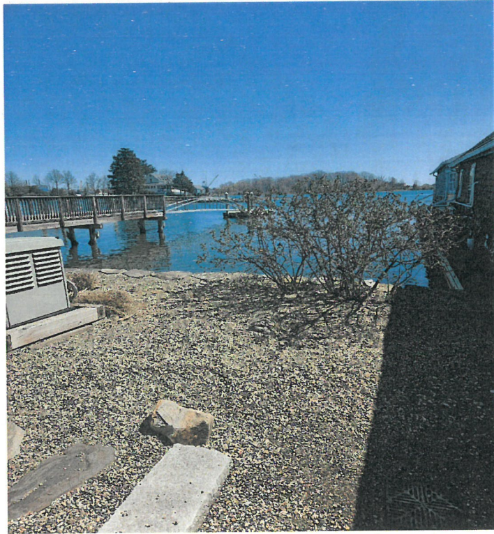
Photo #11: Looking easterly at an existing tree, dock, and stone seawall & shoreline. April 28, 2025
