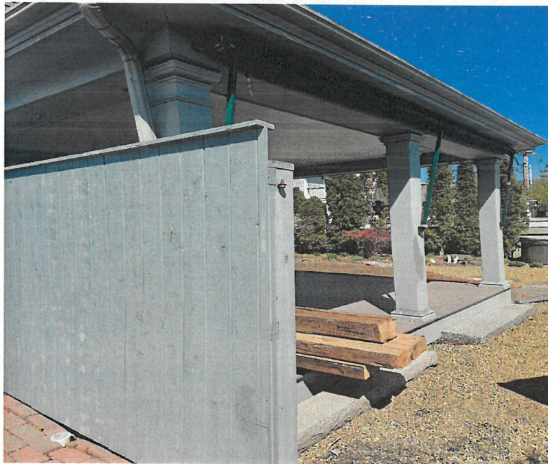
Photo #6: Looking northwesterly at existing porch to be modified into a sun porch April 28, 2025
