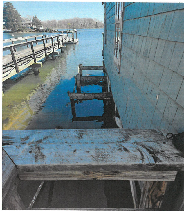
Photo #22: Looking easterly towards wooden supports adjacent to the boathouse. April 28, 2025
