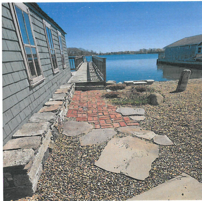
Photo #16: Looking easterly at the brick walkway to be removed leading to the dock which is to remain. April 28, 2025
