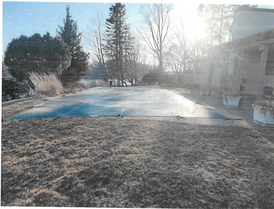
Photo #37: Looking southerly at pool to be replaced & vegetated buffer to be augmented. March 1, 2024
