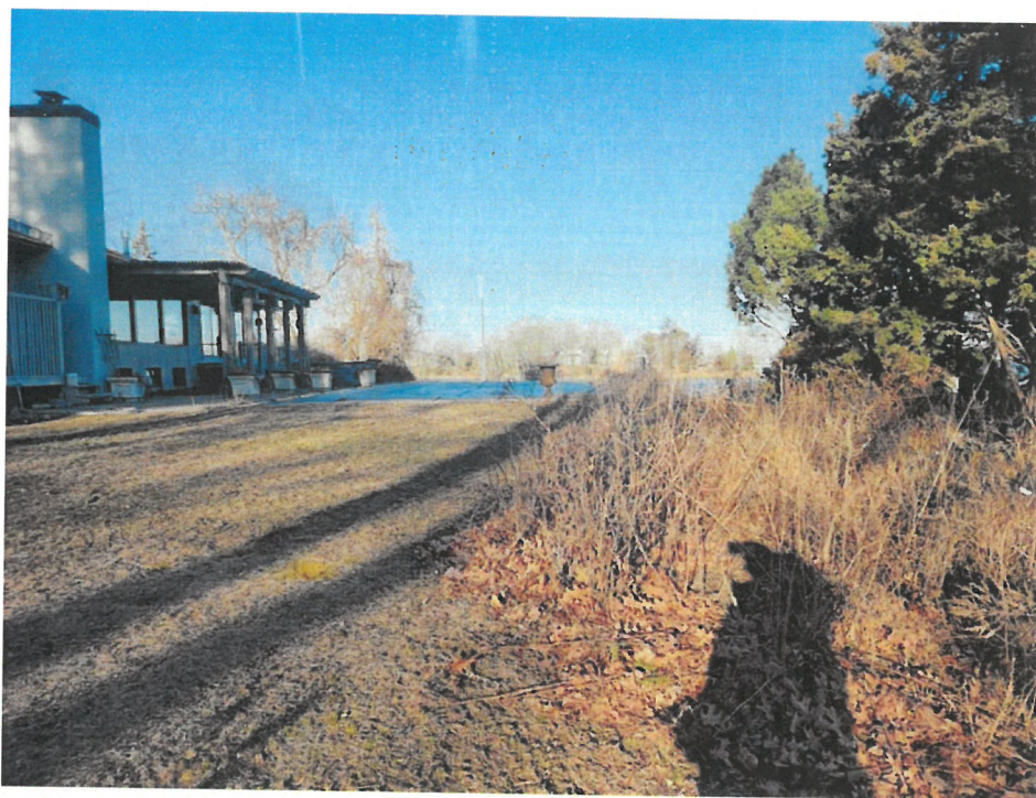
Photo #32: Looking northerly at pool to be replaced & vegetated buffer to be augmented. March 1, 2024
