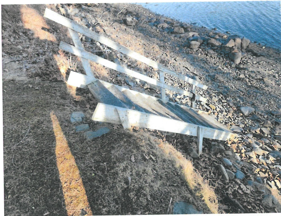
Photo #26: Looking down from lawn/bluff at steps to be replaced. March 1, 2024
