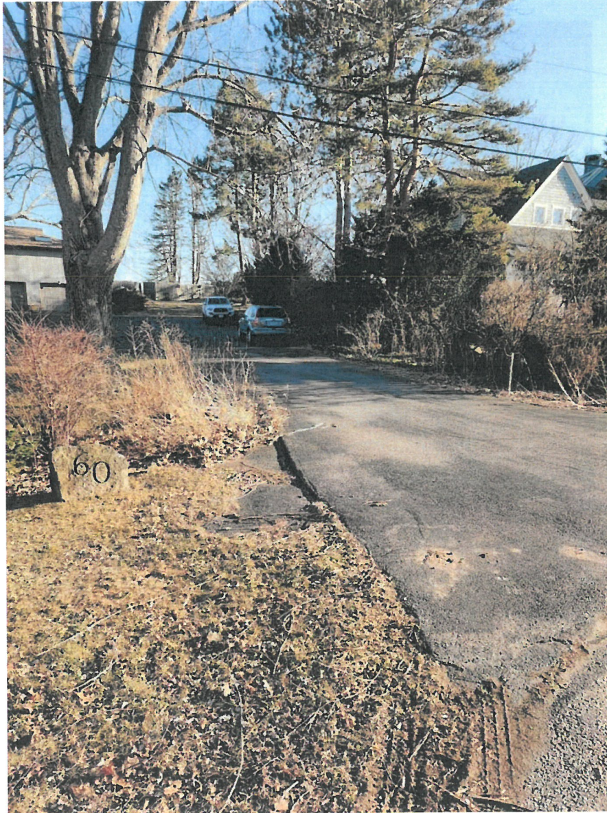
Photo #2: Looking southerly at the driveway to be replaced. March 1, 2024
