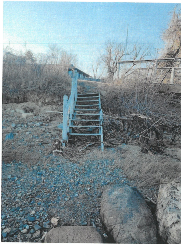
Photo #17: Looking northwesterly at steps to be replaced, shoreline stabilized & vegetated buffer to be augmented. - March 1, 2024
