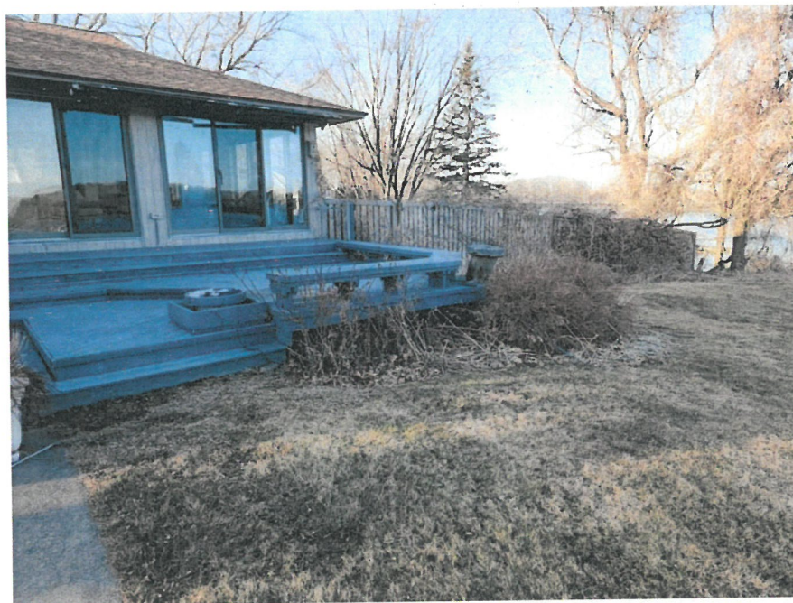
Photo #38: Looking easterly at shoreline and Piscataqua River (resource). March 1, 2024
