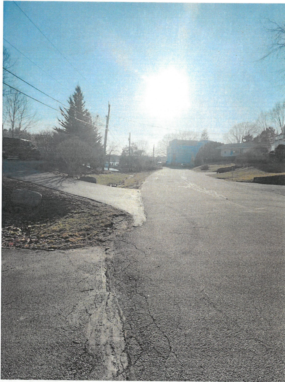
Photo #3: Looking westerly at existing driveway exit on to Pleasant Point Drive. March 1, 2024
