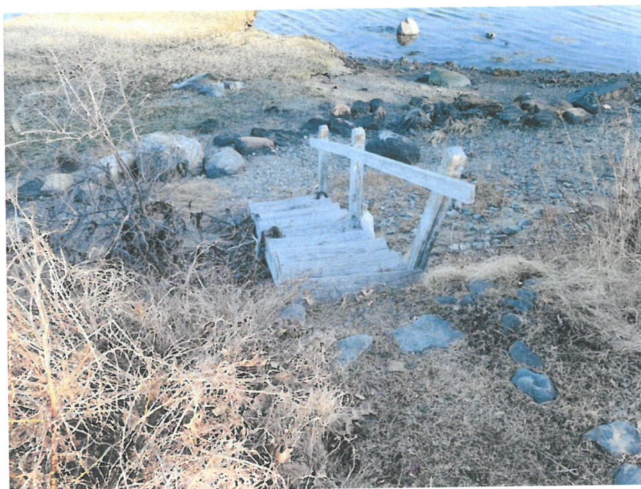
Photo #16: Looking southeasterly at top of steps to be replaced (near existing dock). March 1, 2024
