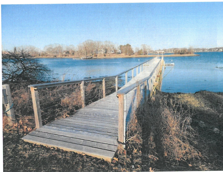
Photo #15: Looking easterly at existing dock to remain and Piscataqua River beyond. March 1, 2024
