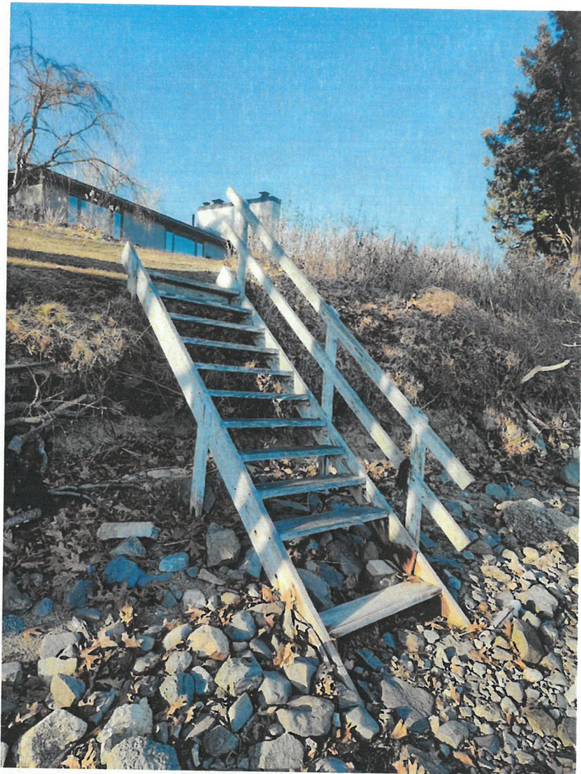
Photo #25: Looking northerly at steps to be replaced. They are above HOTL and will not require foundation support. – March 1, 2024
