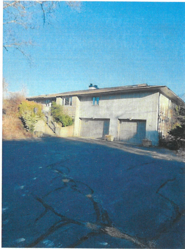
Photo #5: Looking southeasterly at existing driveway and residence to be replaced. – March 1, 2024
