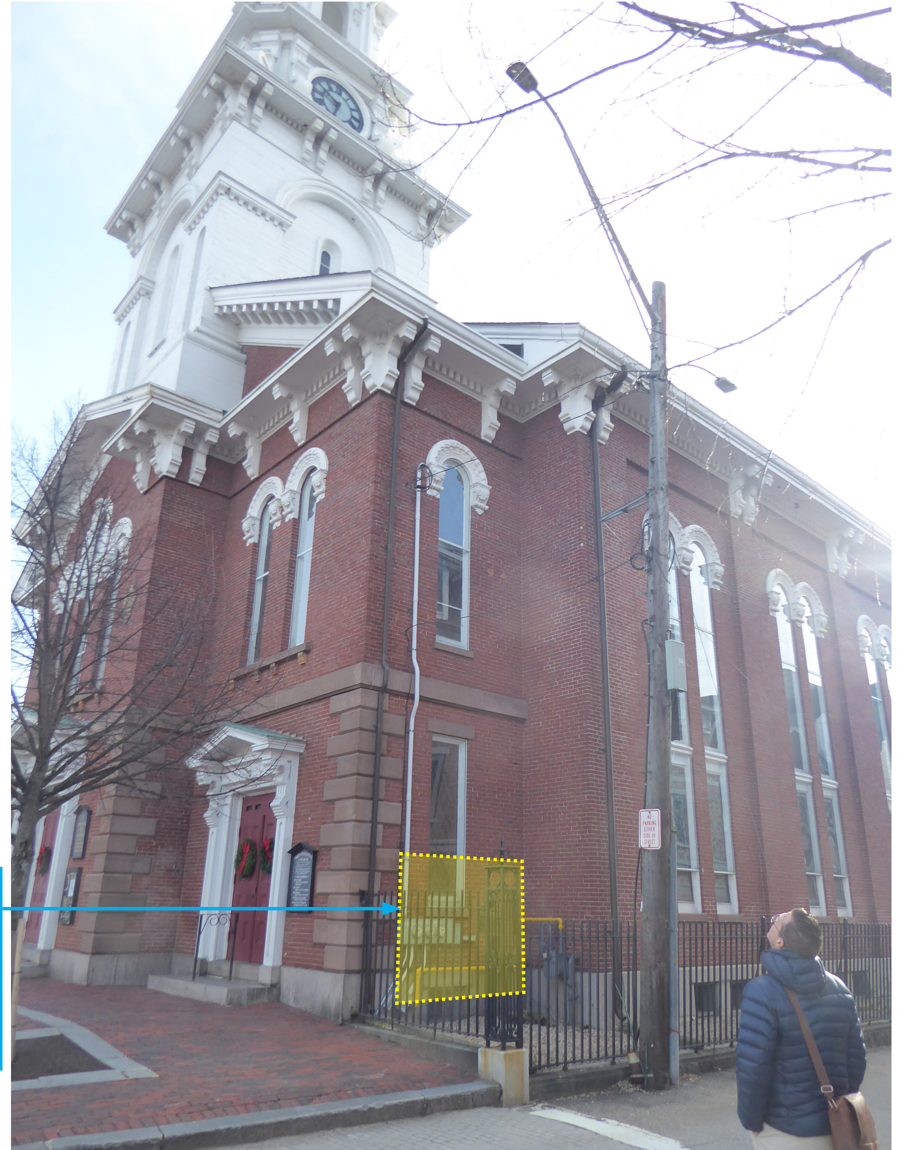
EXISTING VIEW FROM CONGRESS STREET, LOOKING SOUTHEAST
