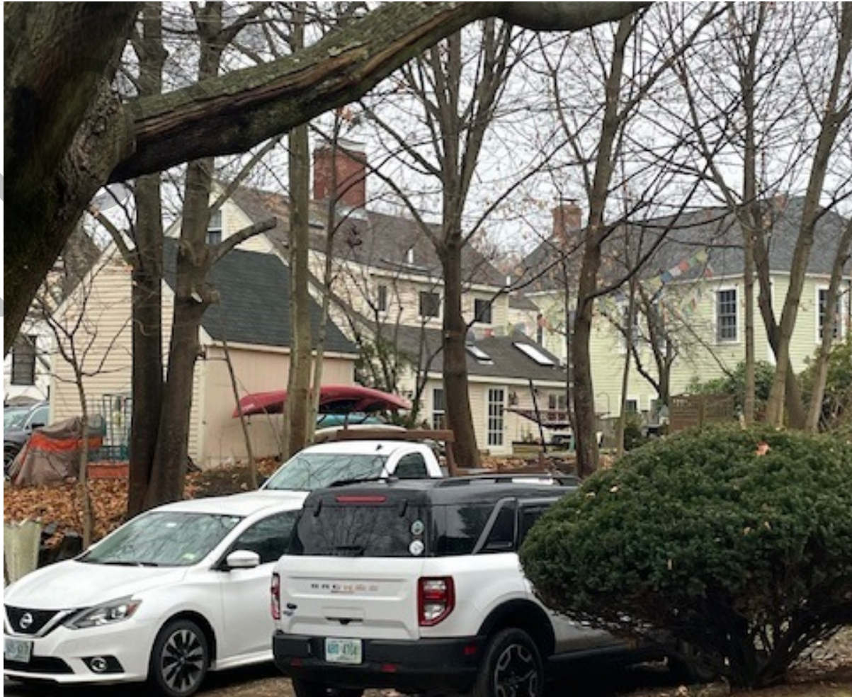
213 SOUTH STREET_SHED DORMER COMING OFF THE BACK
