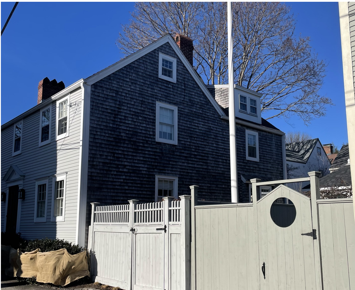
49 HUNKIN STREET_SHED DORMER FACING SIDE
