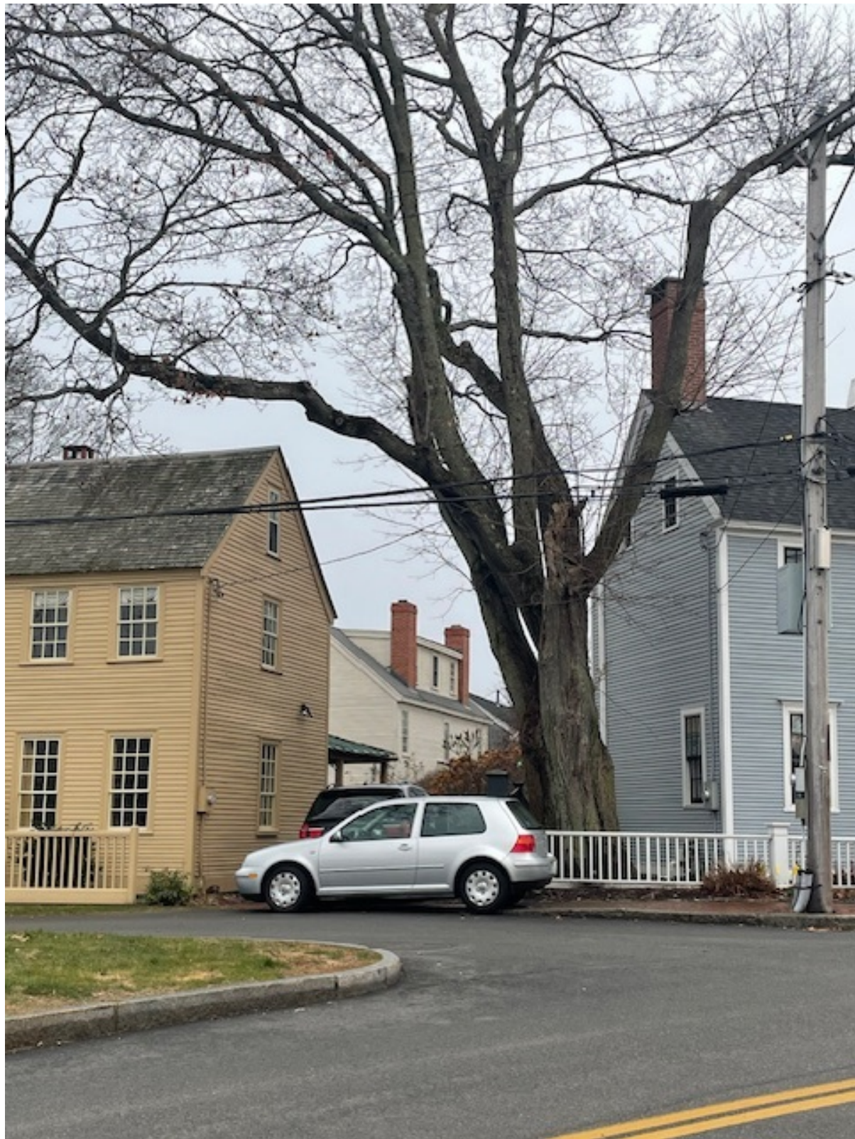
434 MARCY STREET_SHED DORMER STUCK BETWEEN TWO CHIMNEYS
