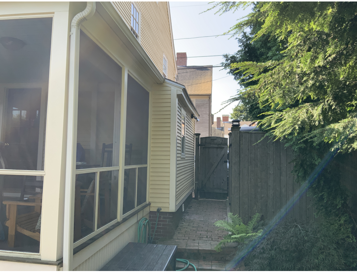
LEFT SIDE REAR SCREEN PORCH & STORAGE AREA
