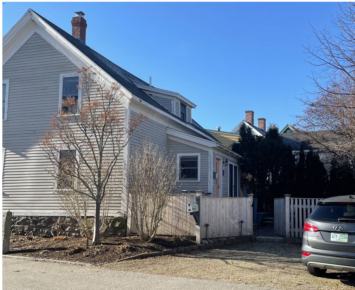
41 SOUTH MILL STREET_SIDE VIEW W/ DORMER
