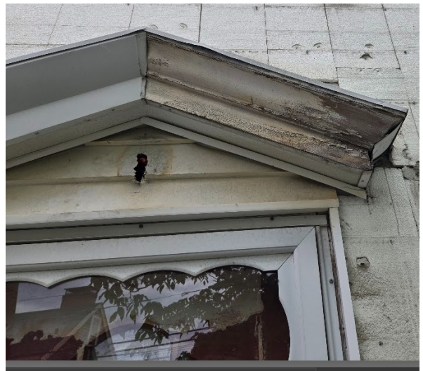
Marcy Street Facing Door Pediment Existing Conditions w/ Metal Cladding Removed
