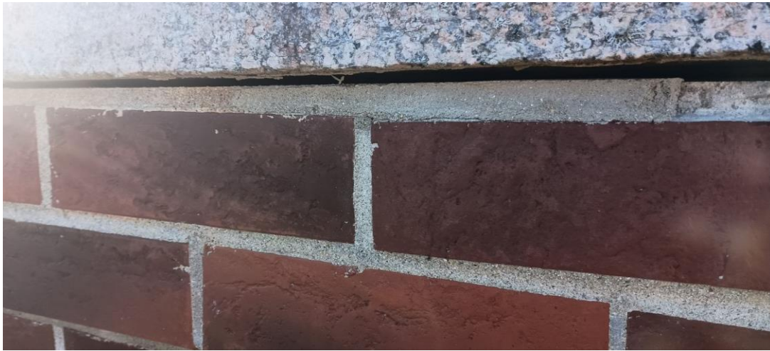
Chimney cap gap before repair
