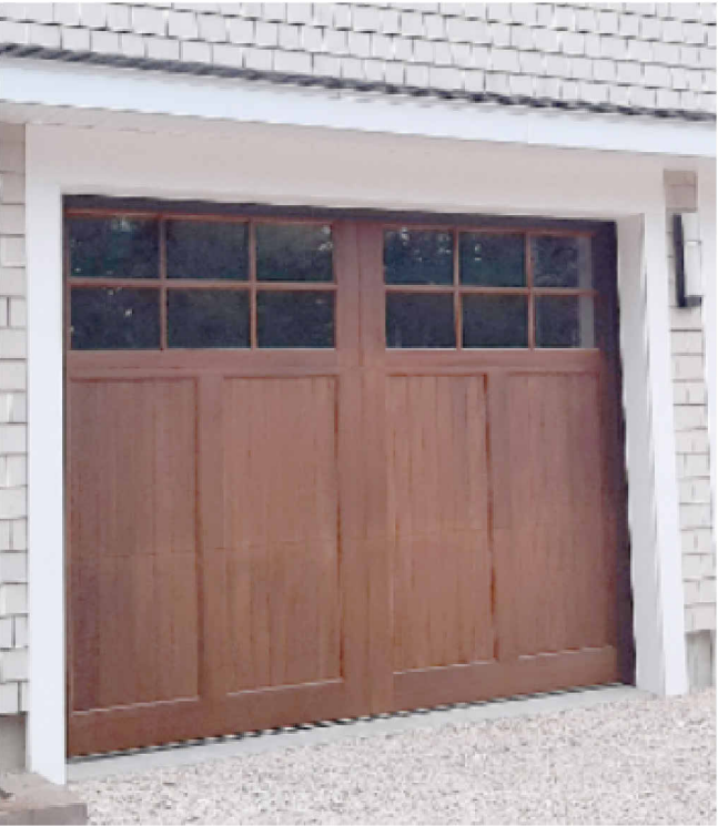
WOOD (CEDAR) PANELED CARRIAGE STYLE OVERHEAD DOOR Manufacturer: RICHARD WILCOX (or equivalent) Series: Landmark™ Rockwood 1" cedar boards on 2" insulated steel panels, SDL 2x6-lite glazing
