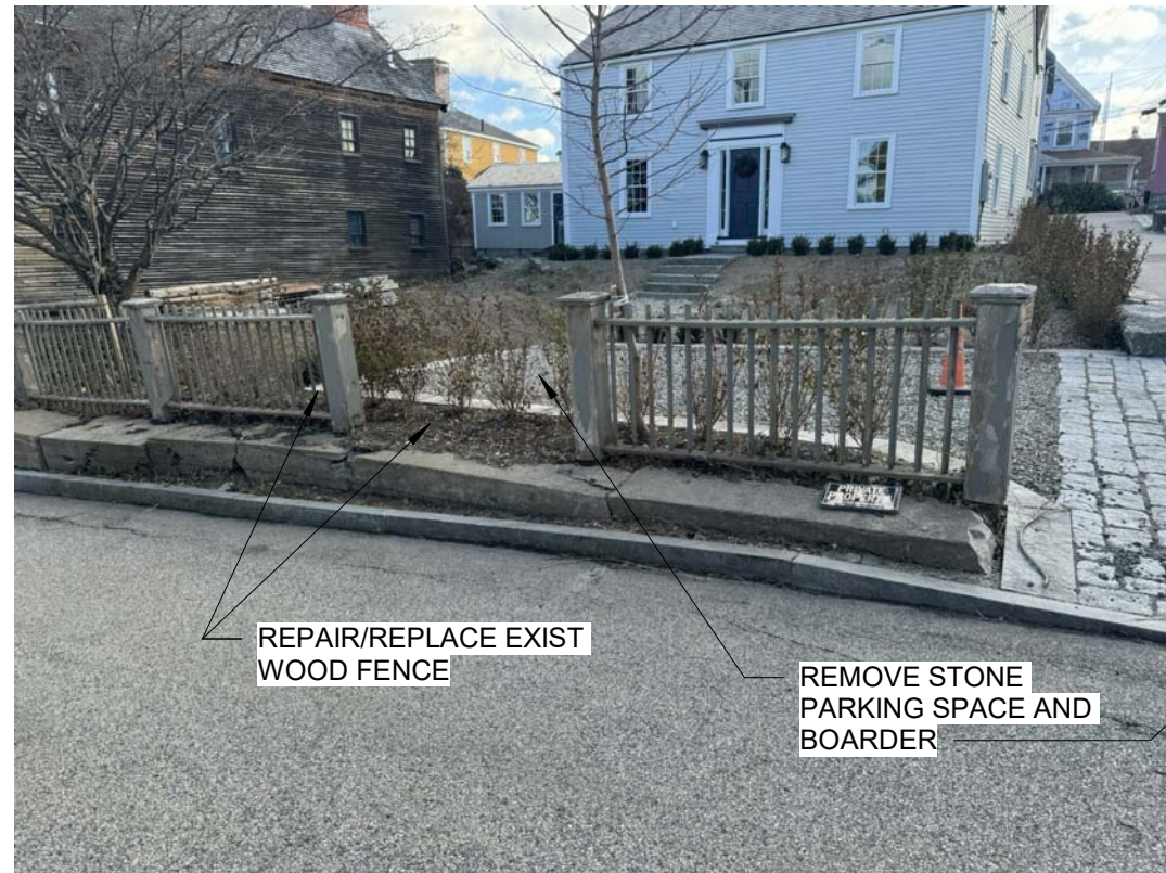
GATES STREET FENCE
