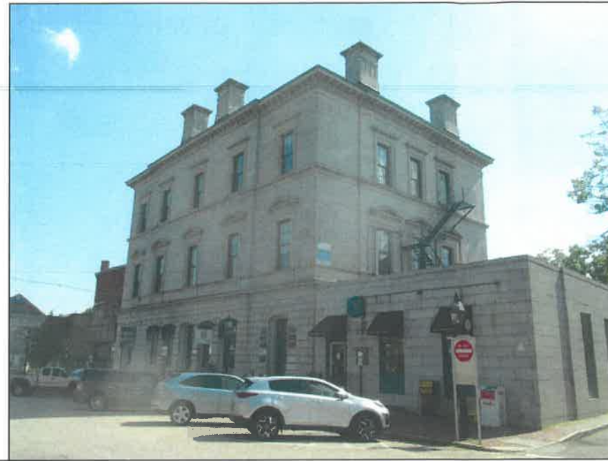
EXISTING NORTH EAST BUILDING CORNER
