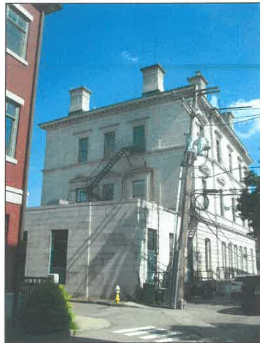
EXISTING NORTH WEST BUILDING CORNER
