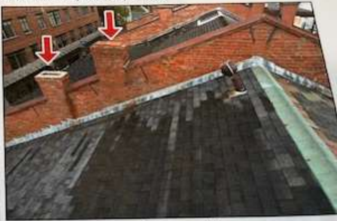
1.0 Item 24(Picture) open chimneys
