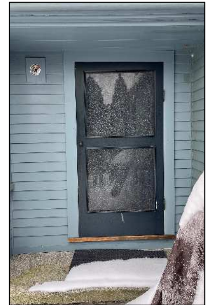
4. BACK LIGHT LOCATION New light to be custom fabricated to match (See Spec)
