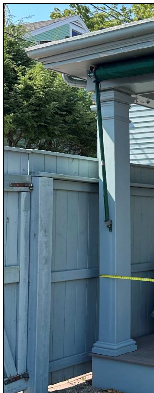
3. COLUMN PROFILE AND EAVE DETAIL To be rebuilt at new Screened Porch
