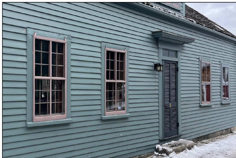
2. DEMONSTRATES INCONSISTENT SILL DIMENSIONS Varies from 1 \frac{3}{4} " to 2 \frac{1}{2} "
