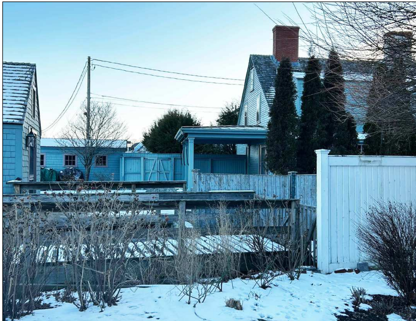
1. EXISTING VIEW FROM SALTER STREET ABUTTERS
