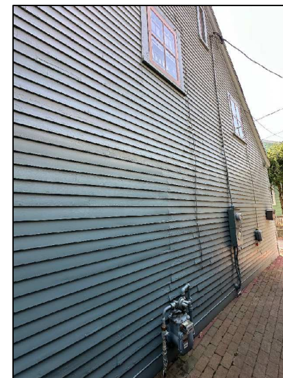
3. DEMONSTRATES INCONSISTENT AGE AND SIDING Siding has been patched in areas of previous window or door openings
