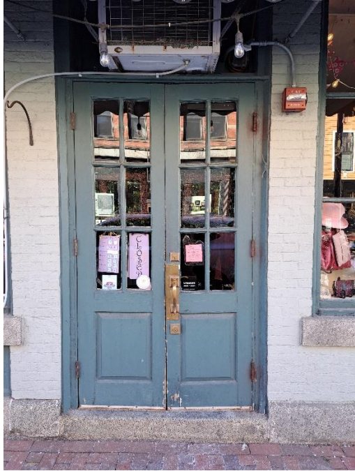
The current doors of 40-42 Market, sagging in towards the middle due to rotted doors & door frame.
