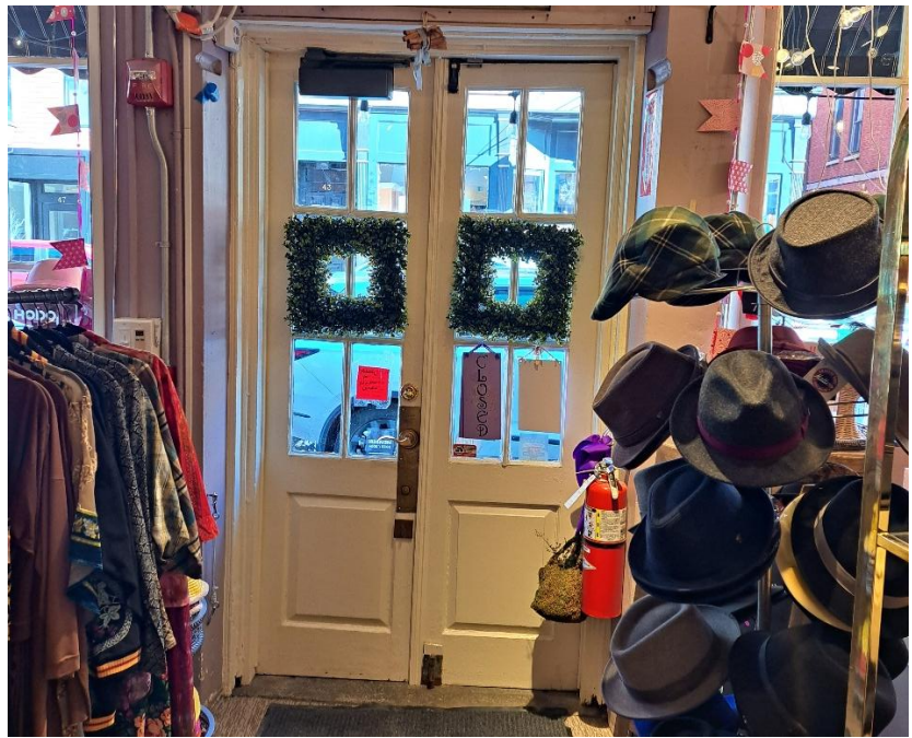
The current doors of 40-42 Market, sagging in towards the middle due to rotted doors & door frame.
