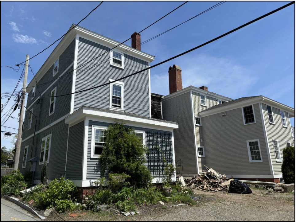
REAR OF BUILDING FROM FRANKLIN STREET
