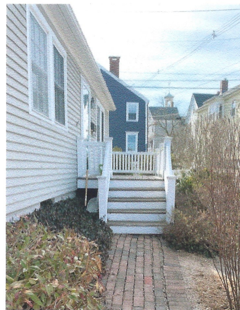
EXISTING FRONT LANDING & STEPS
