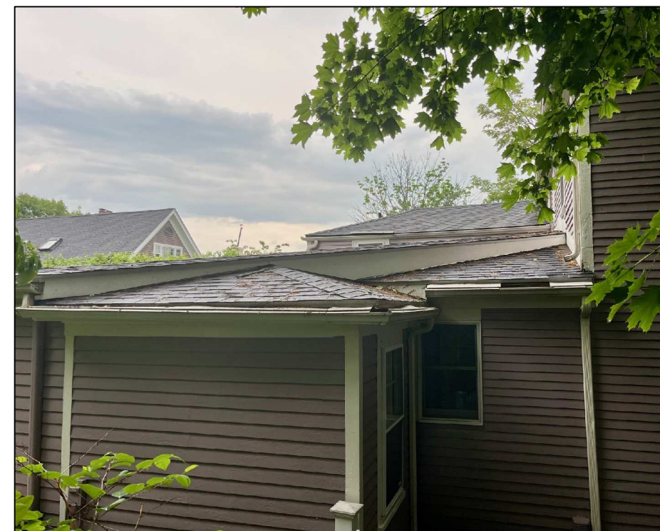
2. Existing Roof Condition
