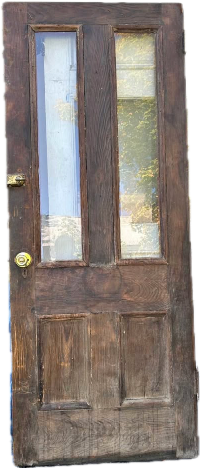
Front porch entry door
