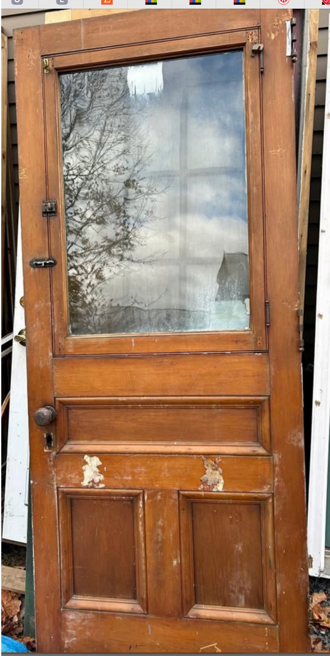
Rear Entry Door
