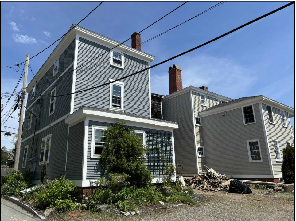
REAR OF BUILDING FROM FRANKLIN STREET
