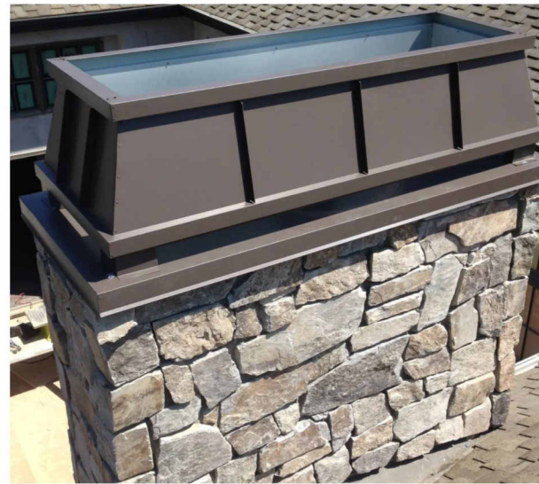
CUSTOM COPPER CHIMNEY SHROUD (FOR GAS FLUE) NATURAL COPPER PATINA CAPO BUILDING SPECIALTIES (OR EQUIV)
