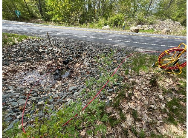
Using Traceable Rodder at Inlet.
