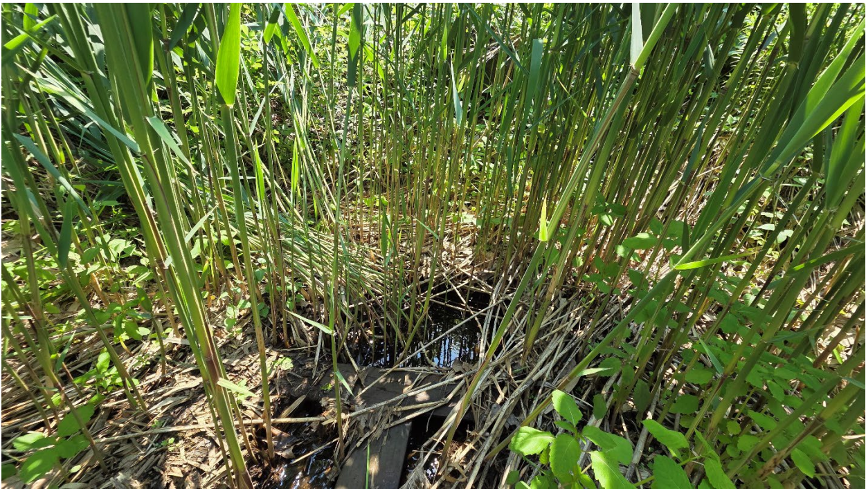
Photo 14 – Liberty Mutual – View of the outlet of Culvert #1 (Photo taken 6/5/2025)
