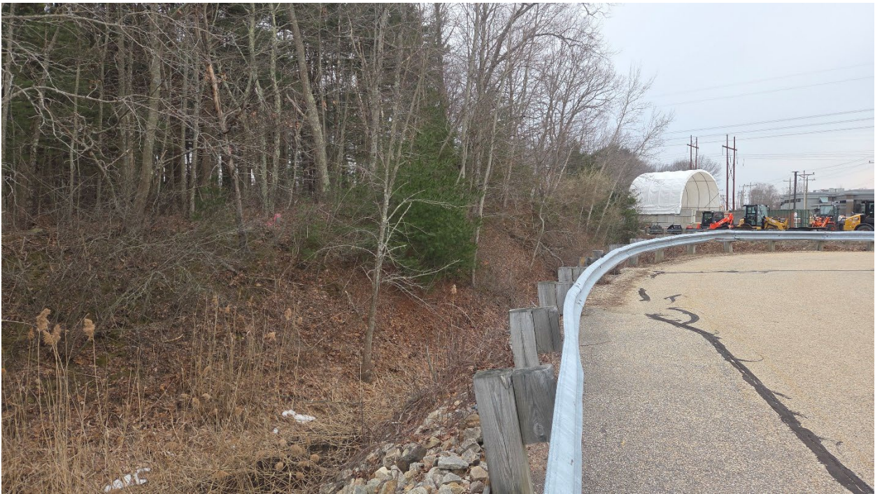
Photo 6 – Liberty Mutual – View looking west along the Stormwater Area along the edge of parking lot (Photo taken 3/20/2026).
